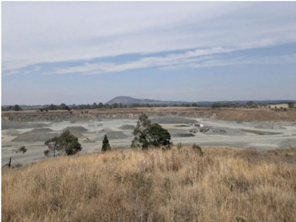
Figure 2 – Image of the existing quarry pit on site (Source: LVIA report)
