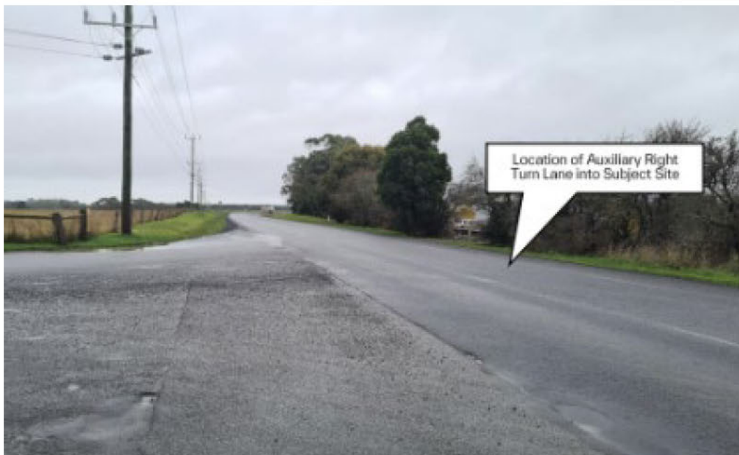
Figure 5 – Entry to site access road (left) where it intersects with Dunnstown-Yendon Road (Source: Road Safety Assessment)
