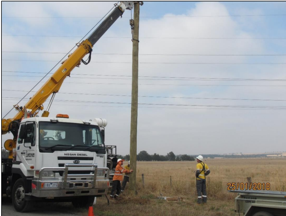
Photograph 3 – Example of a pole being installed via truck crane
