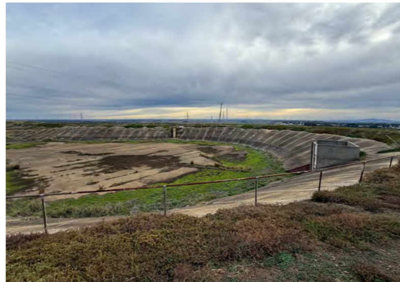
04 concrete lined eastern section of montpellier service basin 1 (not in use)
