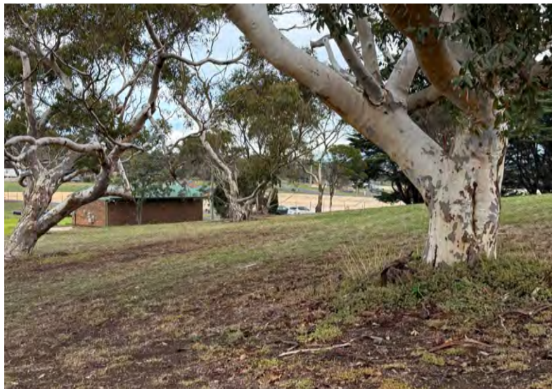
10 view through vegetation to services shed and service basin 2
