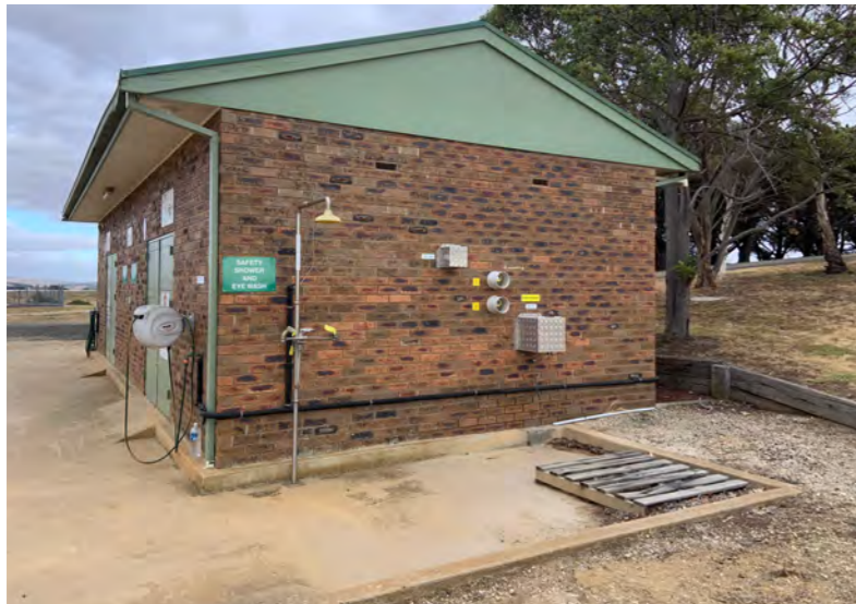
15 south-east view of services shed
