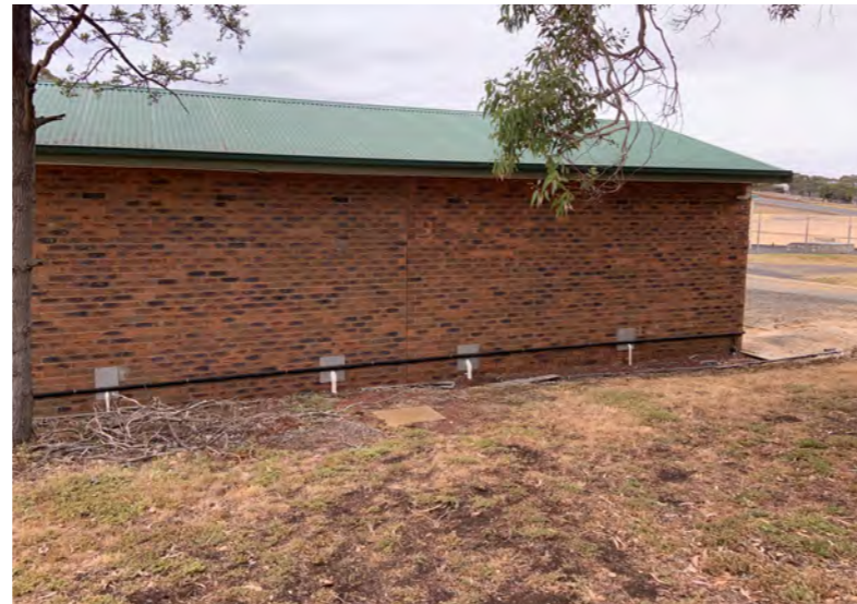
16 north view of services shed
