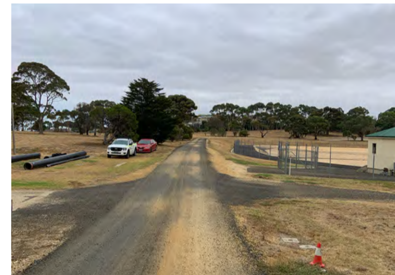
14 existing gravel road beside service basin 2
