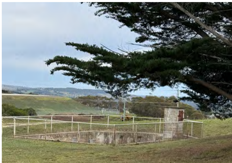
12 existing water distribution pit beneath cypress trees
