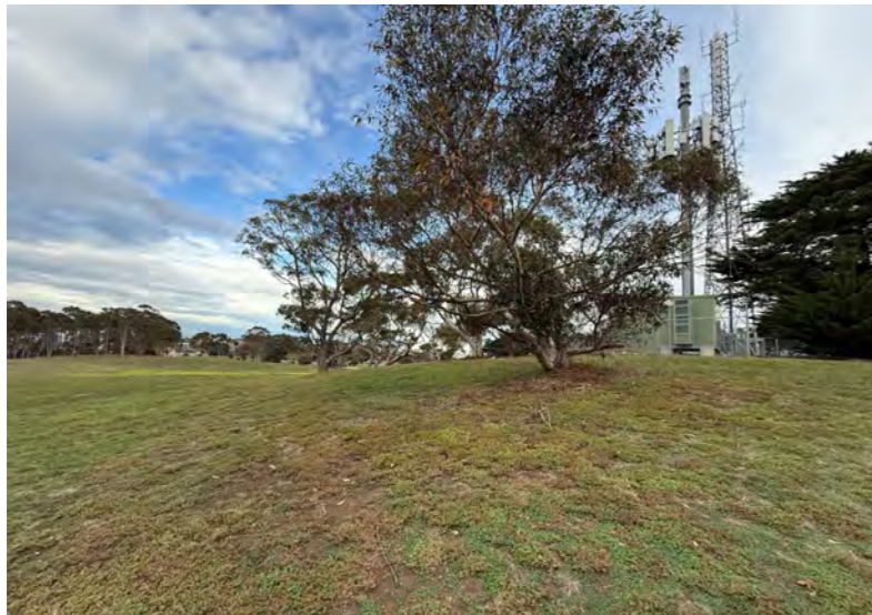
08 view to existing services compound & telecommunications tower
