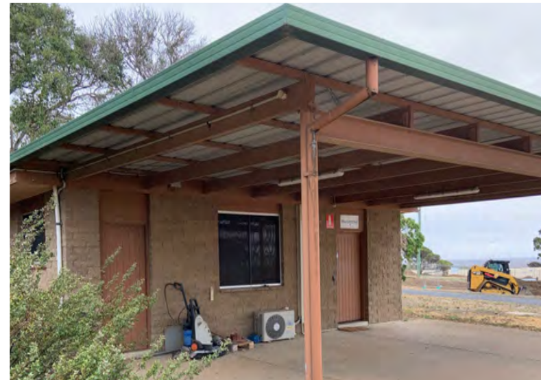
09 existing site office with canopy
