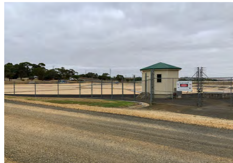
13 services basin 2 and associated site infrastructure
