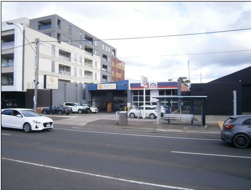
Adjoining development to south of subject site
