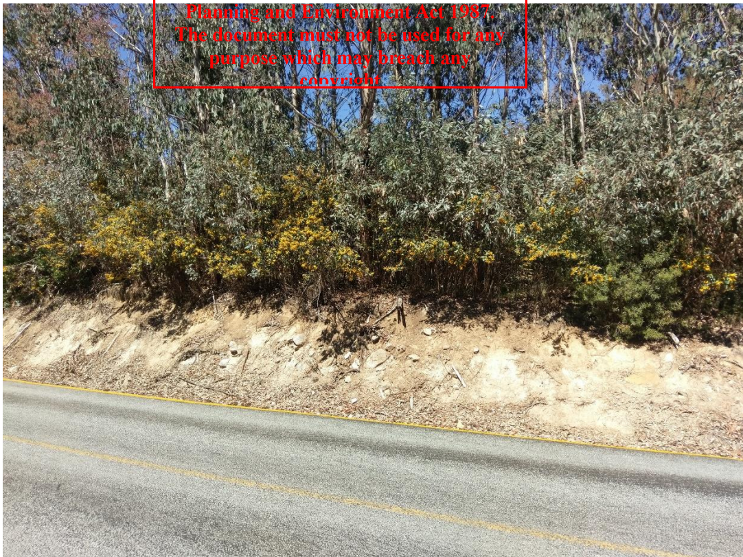
Photograph 4 Low cut slope height (approximately 2-3m) along Bogong High Plains Road to the east of the site. Vegetation shows no sign of movement
