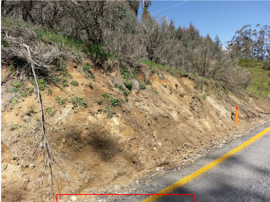
Photograph 3 Cut slope below the north east of the site in natural material (probably extremely weathered rock)
