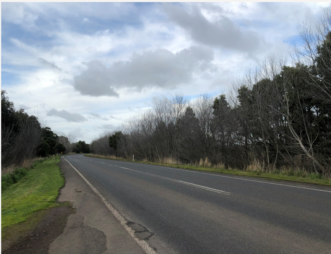
Figure 37 - Viewpoint 6 at Cobden-Terang Road on the northern boundary of the site
