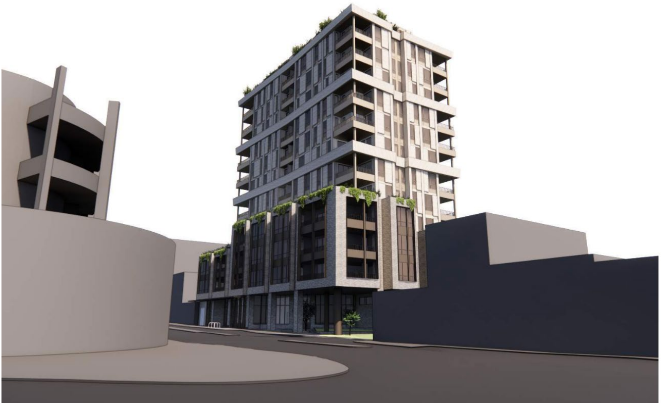
Figure 9 – view from northern footpath of Glenhuntly Road (source: CBG)
