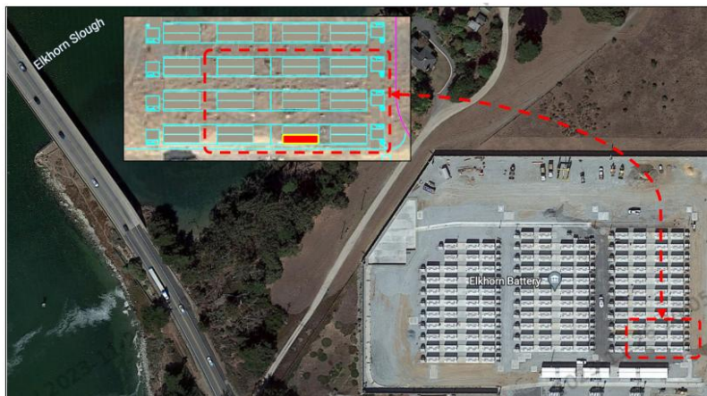
Figure 28: Overview of Elkhorn BESS and Megapack on fire.
