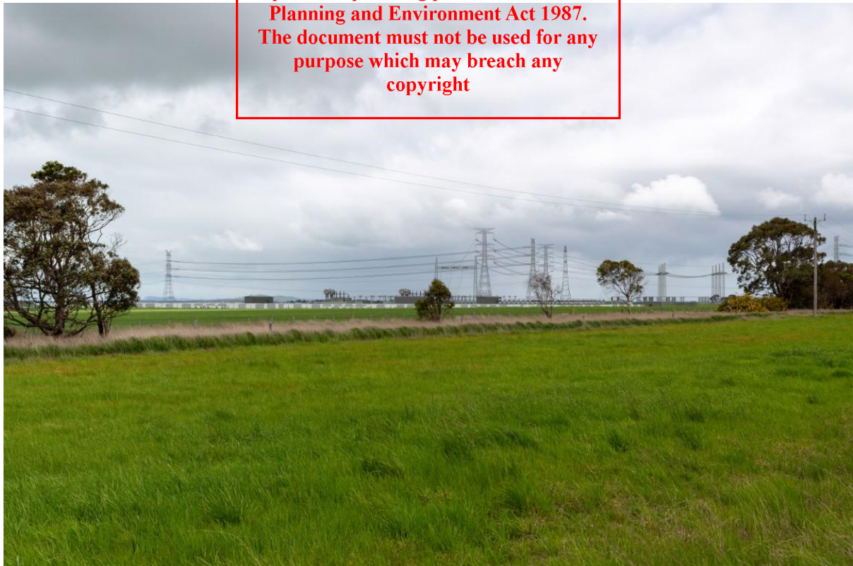
Figure 41 – VP1 – Photomontage - View south southeast from Darlington-Terang Road to the Project – at completion of construction.
