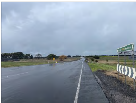
Figure 7: Hamilton Highway - View Northeast
