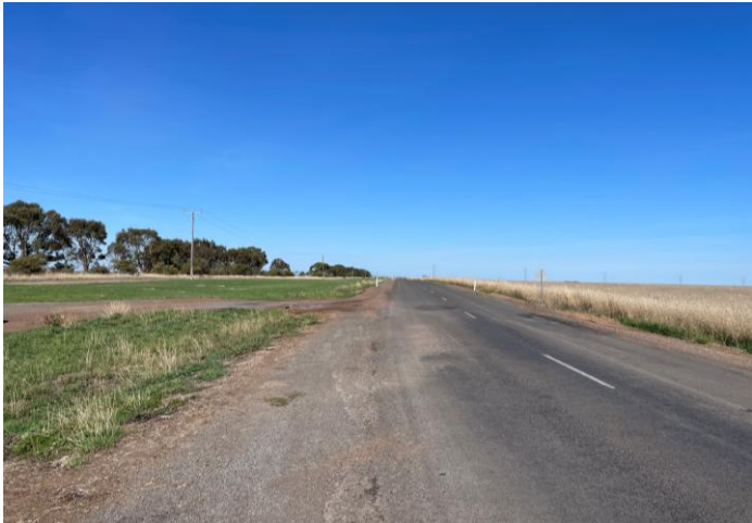
Figure 9: Existing emergency and farm access to the site (west), viewed from Darlington-Terang Rd.
