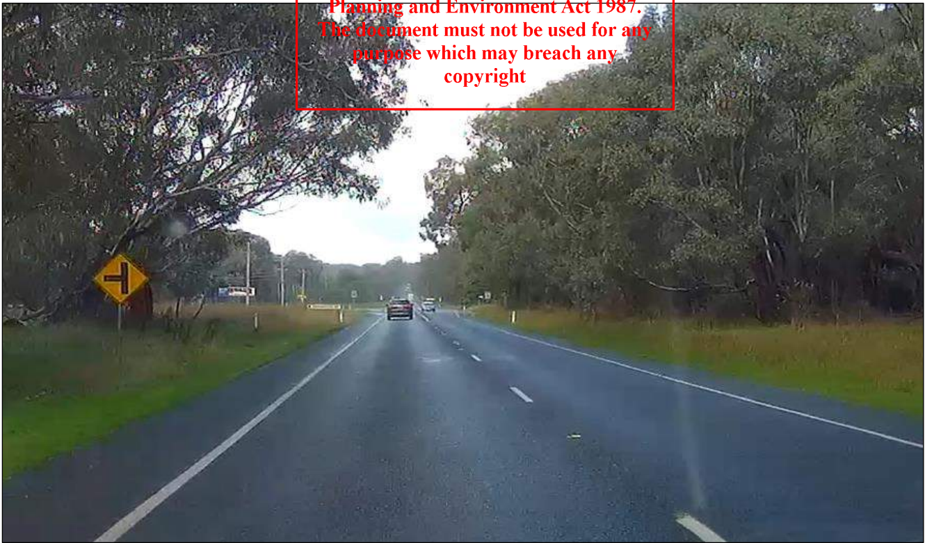
Figure 4: Kiewa Valley Highway facing southeast
