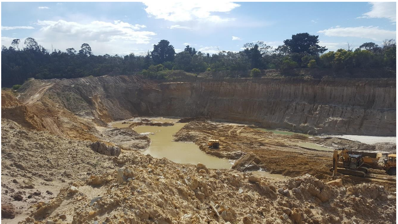
FIGURE 2.1: EXISTING EXCAVATION (FOREGROUND) AND 60 VALLEY ROAD PROPERTY (BACKGROUND)
