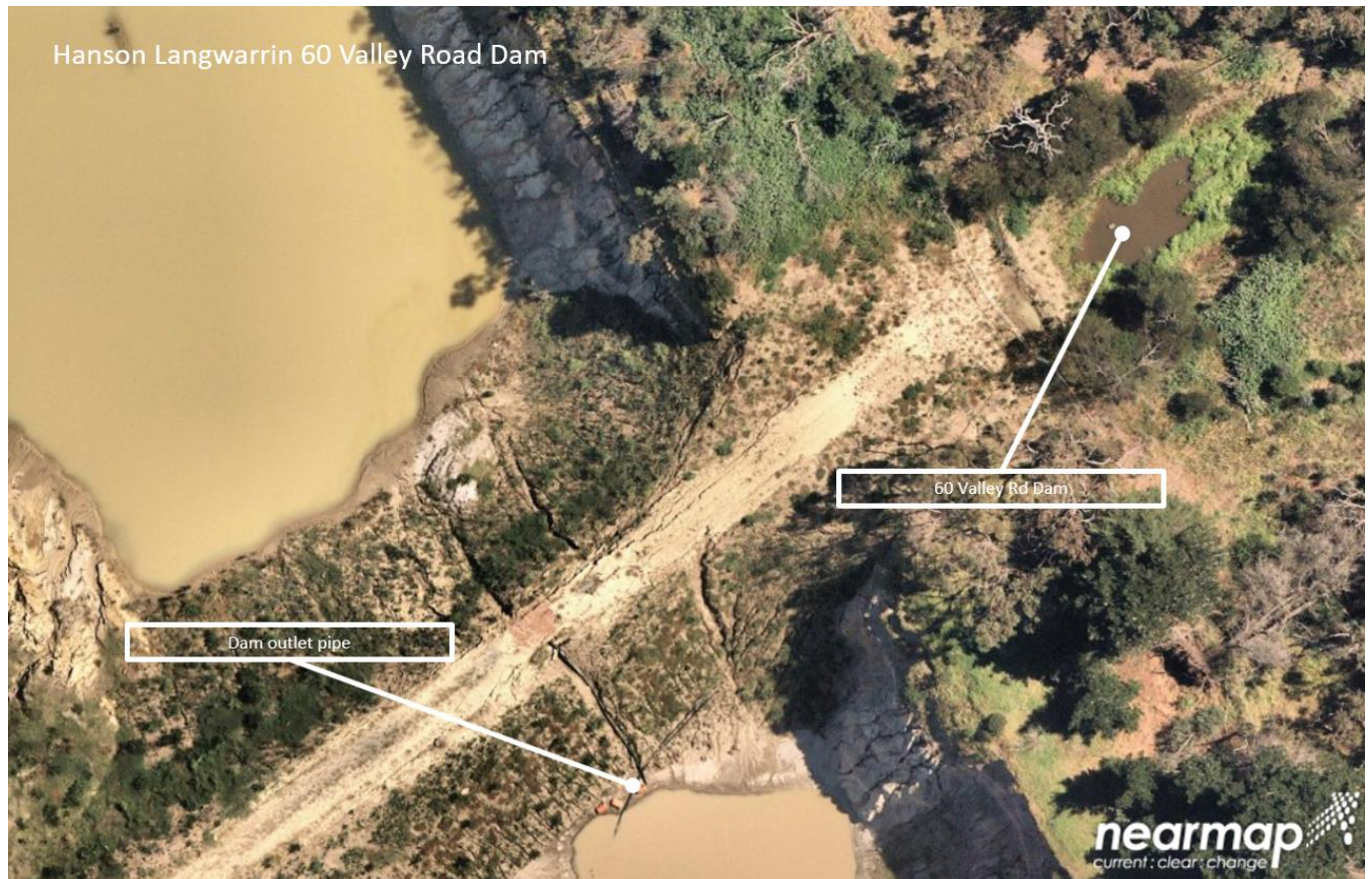
FIGURE 1.2: CURRENT CONFIGURATION OF THE DAM, AFTER REINSTATEMENT RESULTING FROM AN EROSION EVENT IN AUGUST 2019
