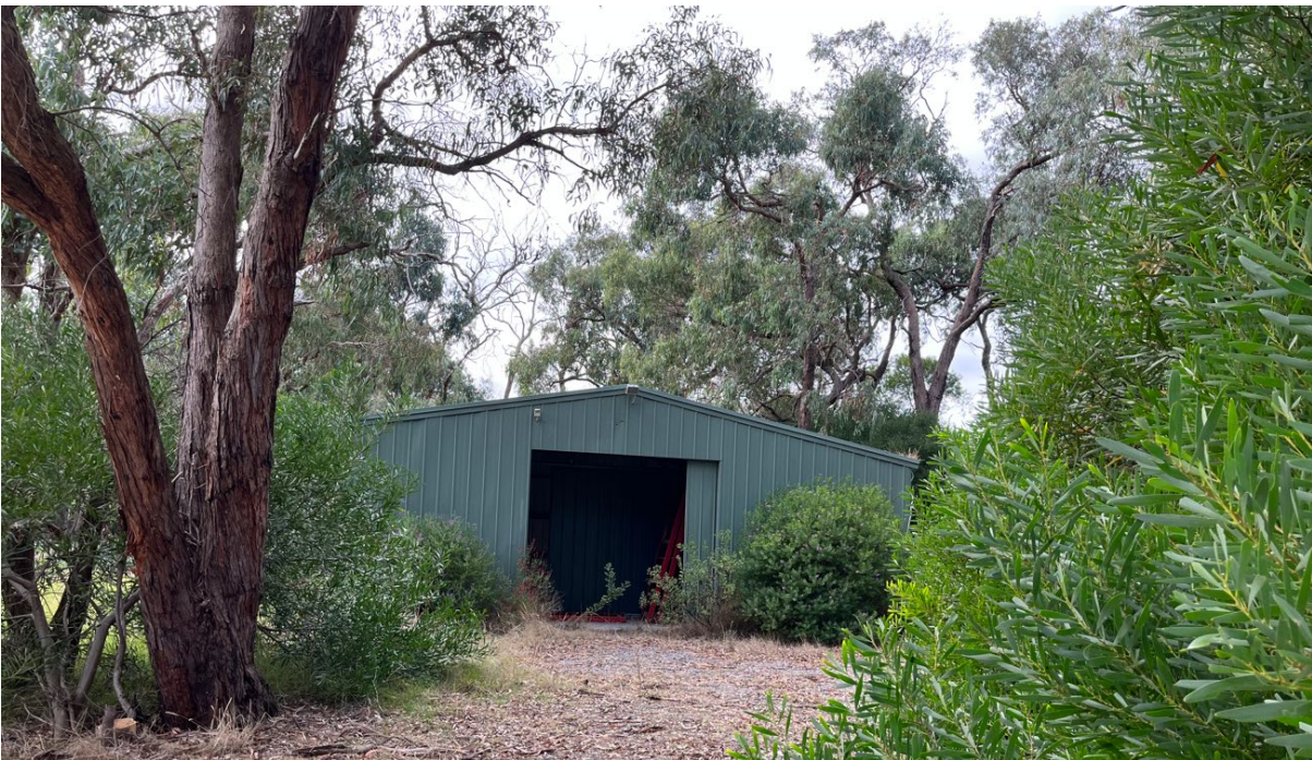
Figure 3 Shed on the Subject Site
