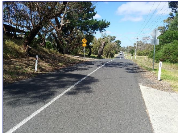
Figure 24: Valley Road – view west
