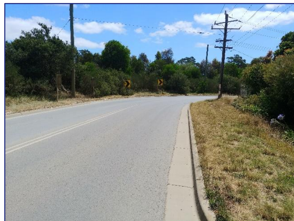
Figure 18: Quarry Road – view northwest (towards bend south of Central Crossover)
