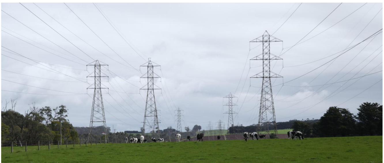
Figure 7-7 Landscape Character Unit 4 – Infrastructure example
