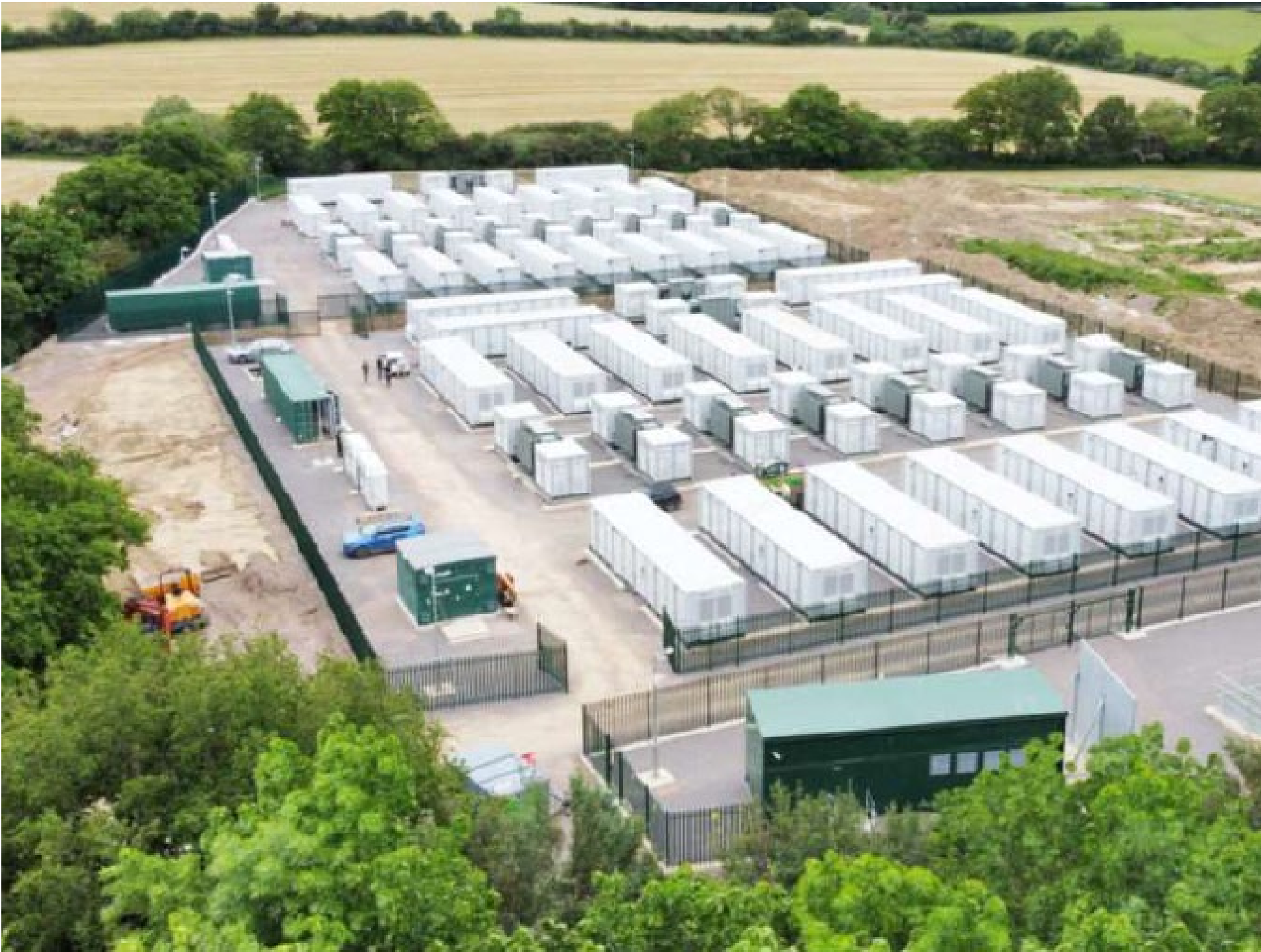
Figure 3-2 Typical BESS layout
