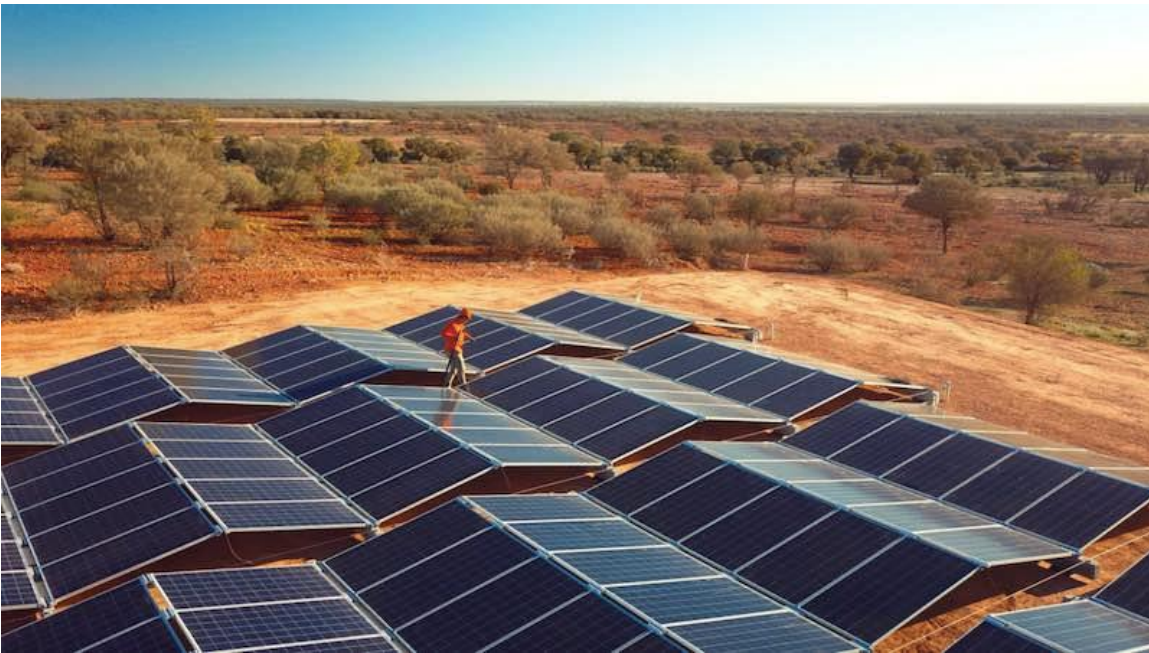
Images 3 & 4: The PEG and 5B Maverick have low ground clearance and require harsher vegetation management than the SMS system.
