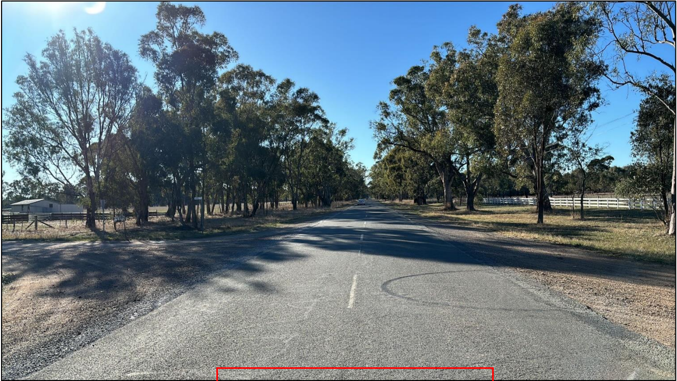
Figure 7: Baddaginnie-Benalla Road facing northeast adjacent to the intersection with Carrol Road (to the left) and Forshaw Road
