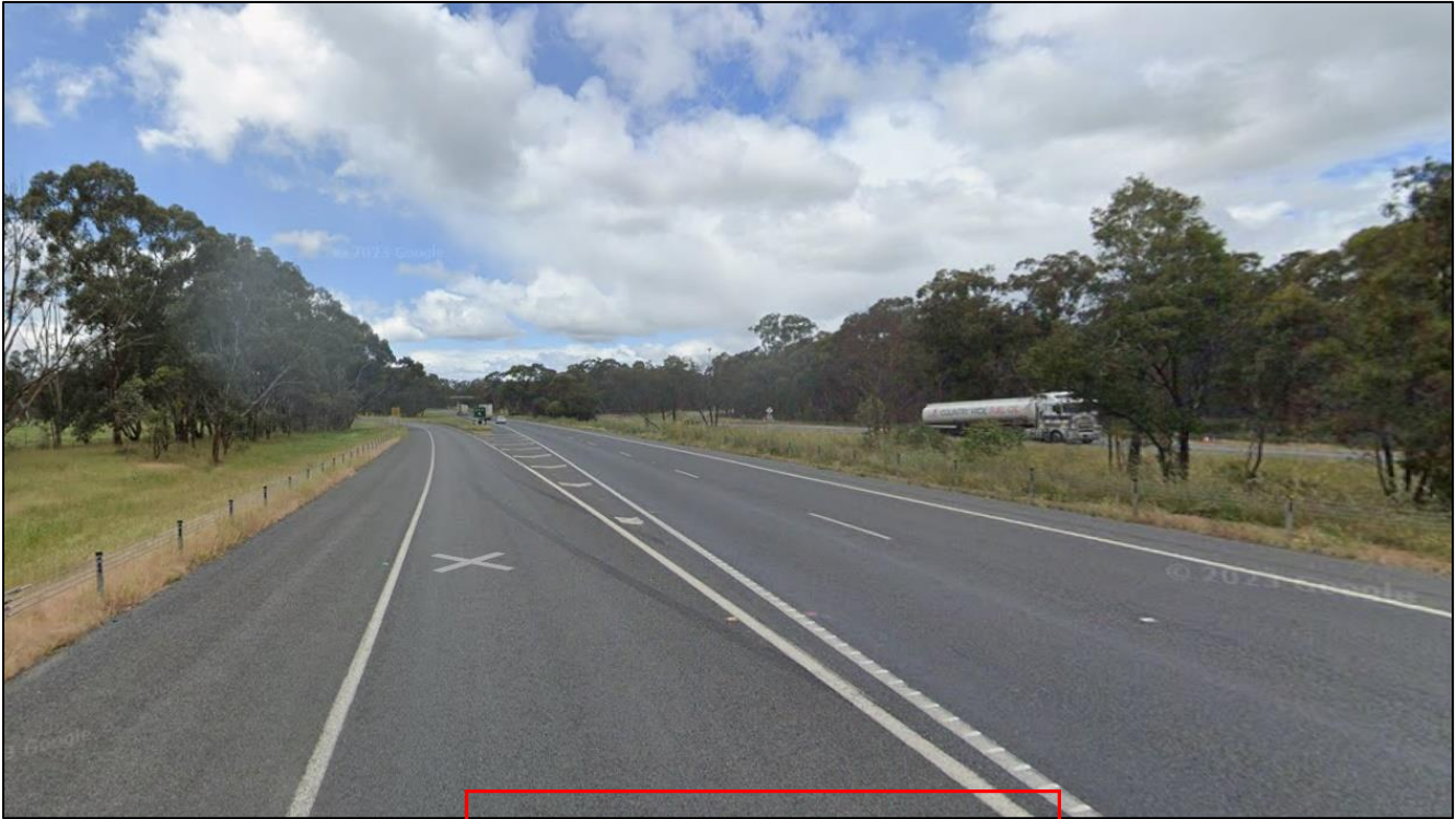
Figure 3: Hume Freeway northbound at the Mansfield Road off-ramp – Source: Google Streetview
