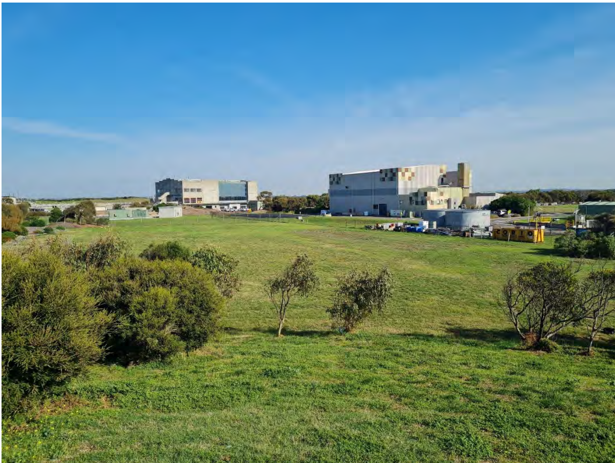
Plate 1 South east corner of Activity Area, facing west
