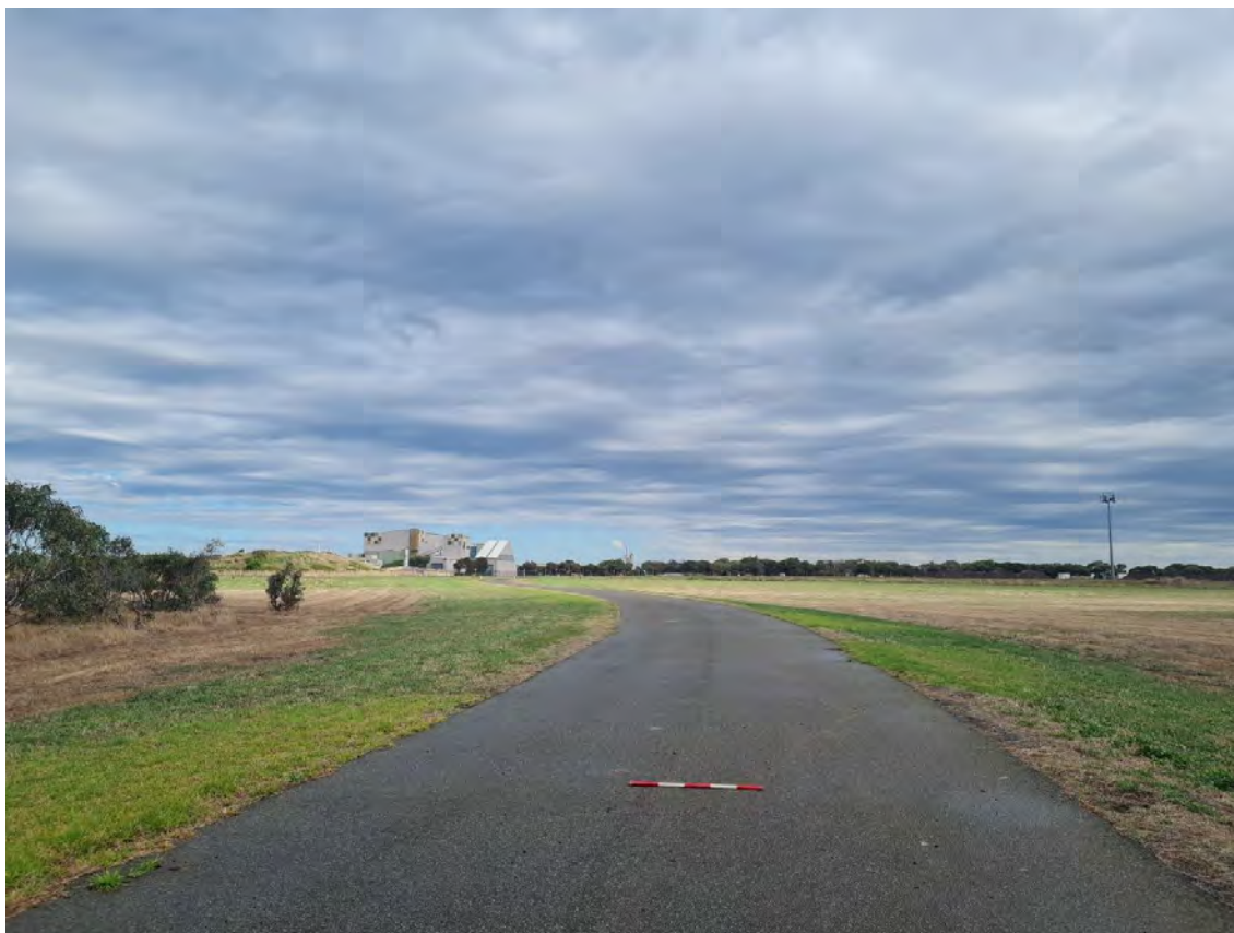
Plate 73 Northern most access road, facing west. (R. Stewart 26.04.2023)
