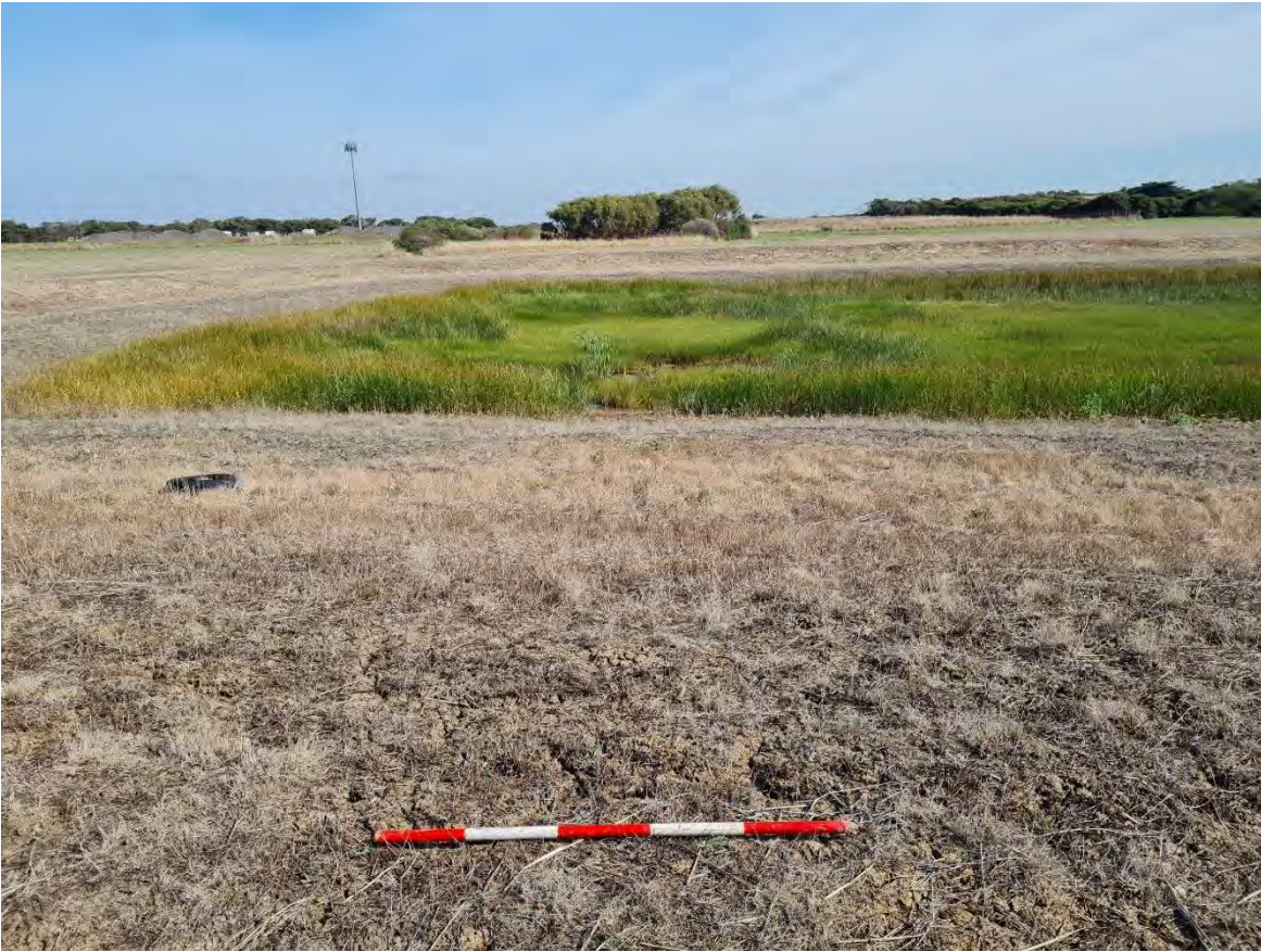
Plate 70 Top of dam wall facing west (R. Stewart 26.04.2023)
