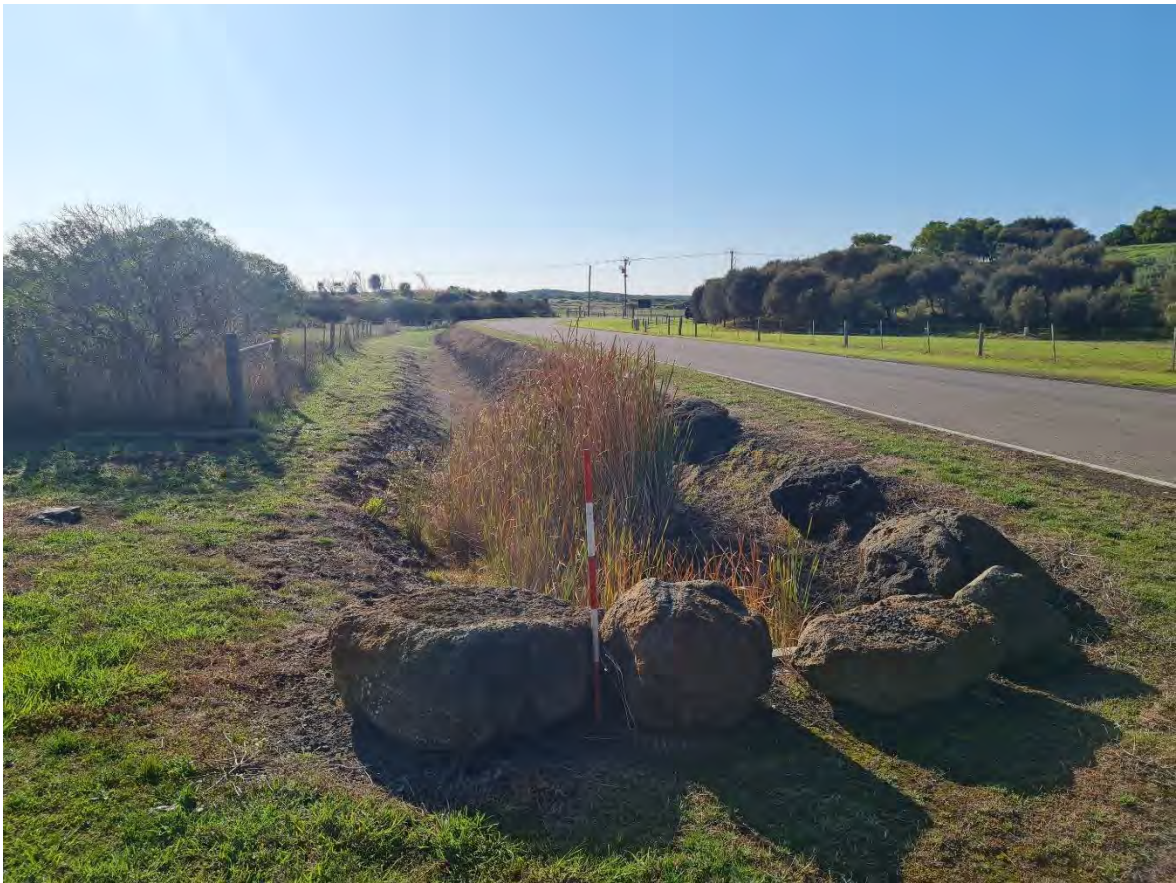
Plate 24 Drain cut adjacent to access road, facing east (R. Stewart 26.04.2023)
