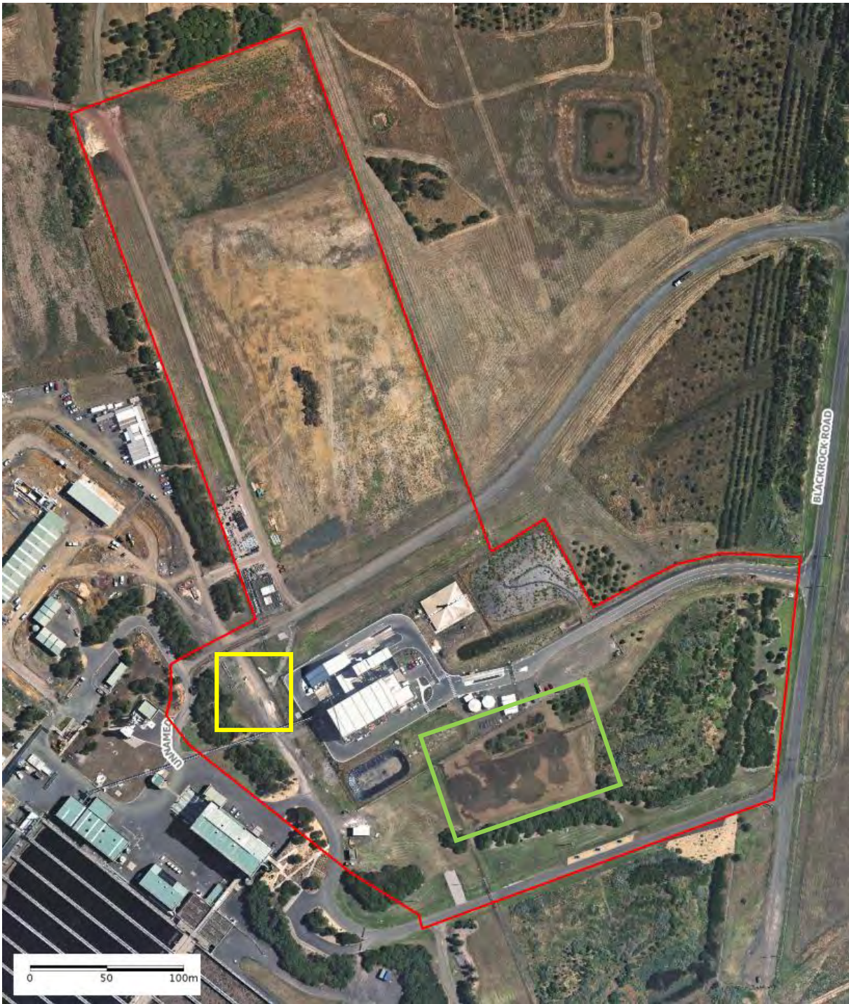
Plate 11 2012 aerial image (DEECA, 2023), Activity Area in red, utility installation areas in yellow, and old carpark in green
