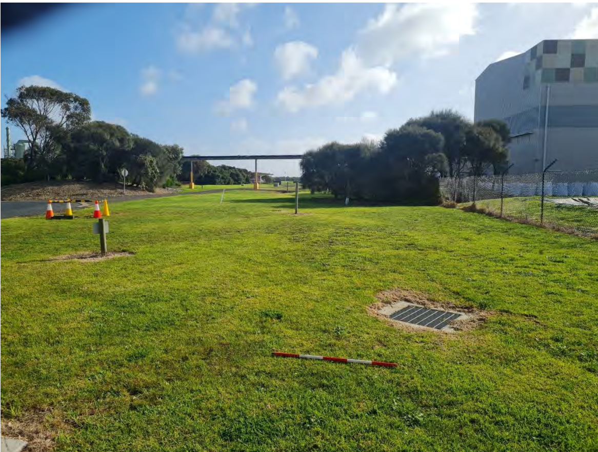
Plate 40 Facing north, utility connection and gravel access road, BTP to east (R. Stewart 11.07.2023)
