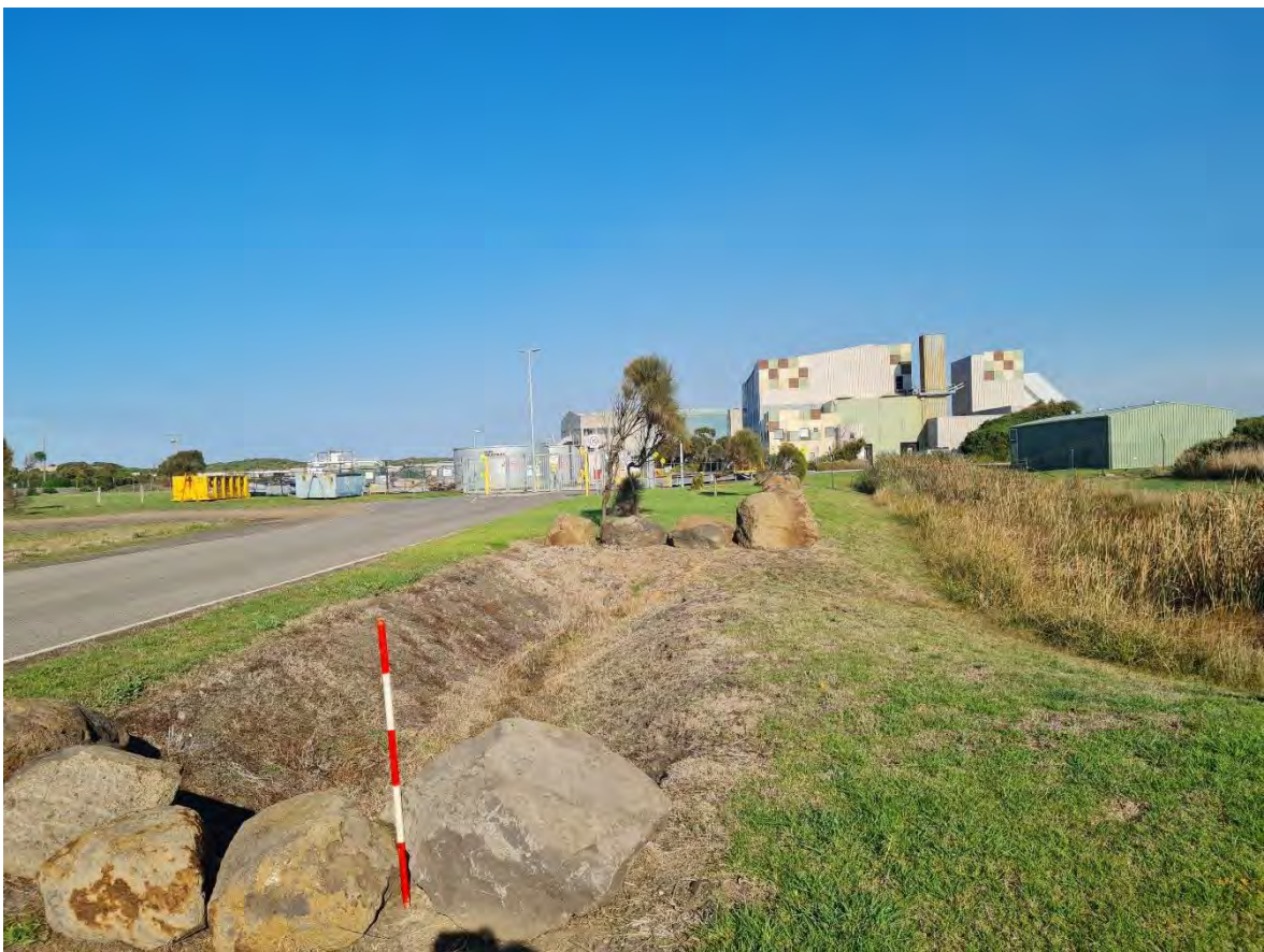
Plate 25 Drain cut adjacent to swale, facing west towards BTP (R. Stewart 26.04.2023)
