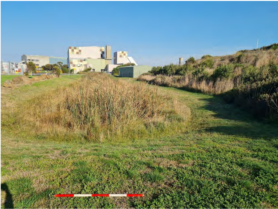
Plate 26 Swale drain, facing west towards BTP (R. Stewart 26.04.2023)
