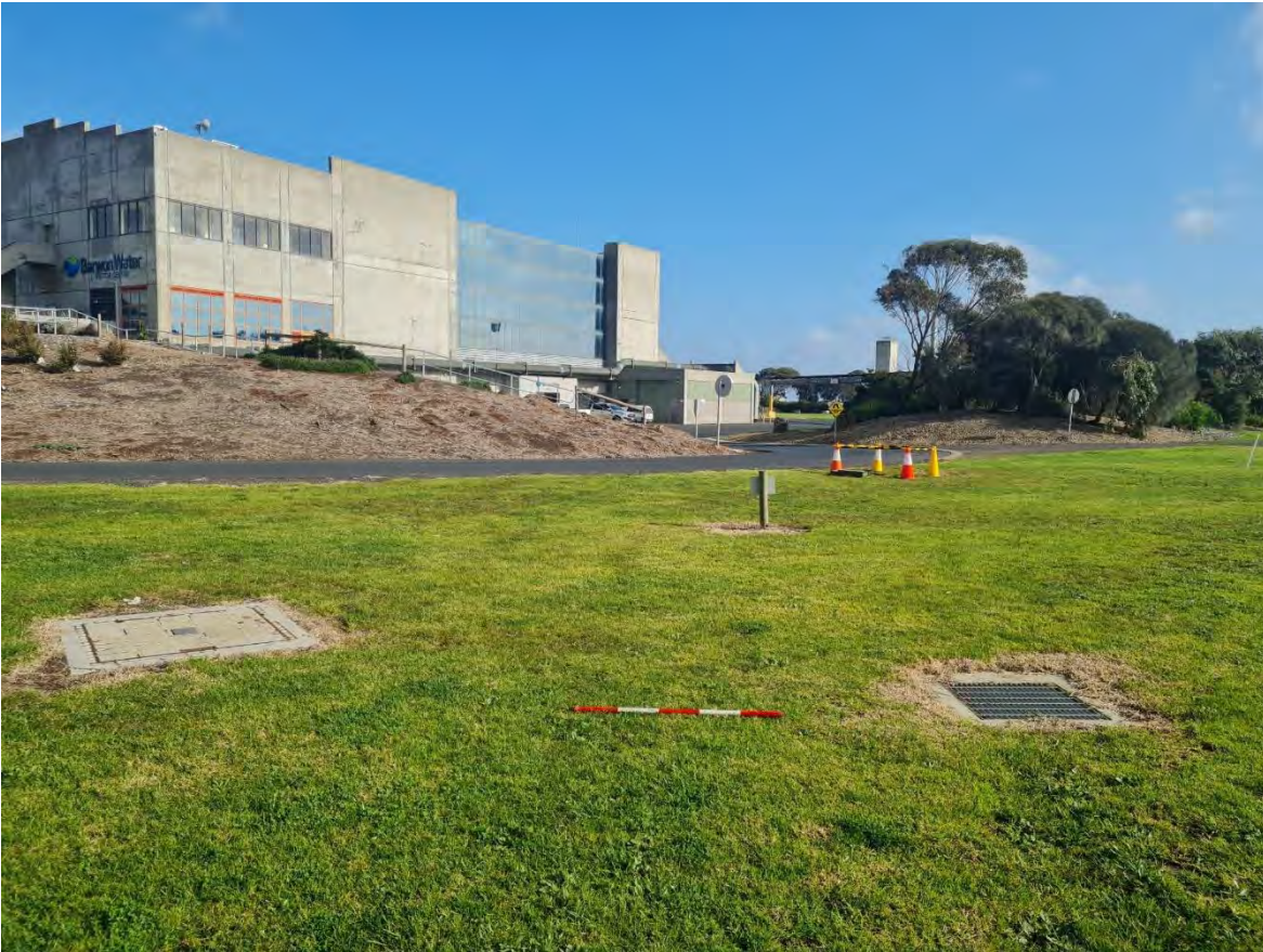
Plate 39 Facing west towards visitors centre, with utility connections (R. Stewart 11.07.2023)
