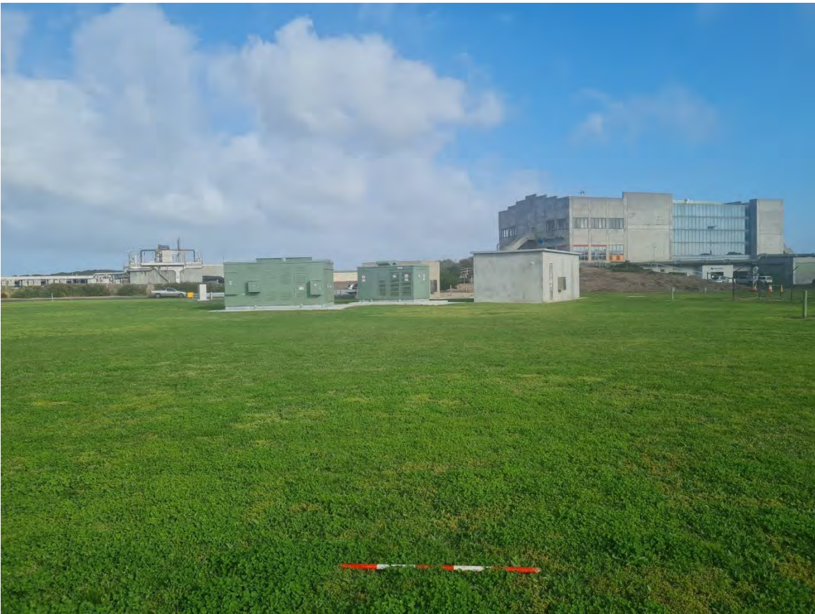
Plate 29 Southwest corner of Activity Area, facing west toward BW site office, with substation in foreground (R. Stewart 11.07.2023)
