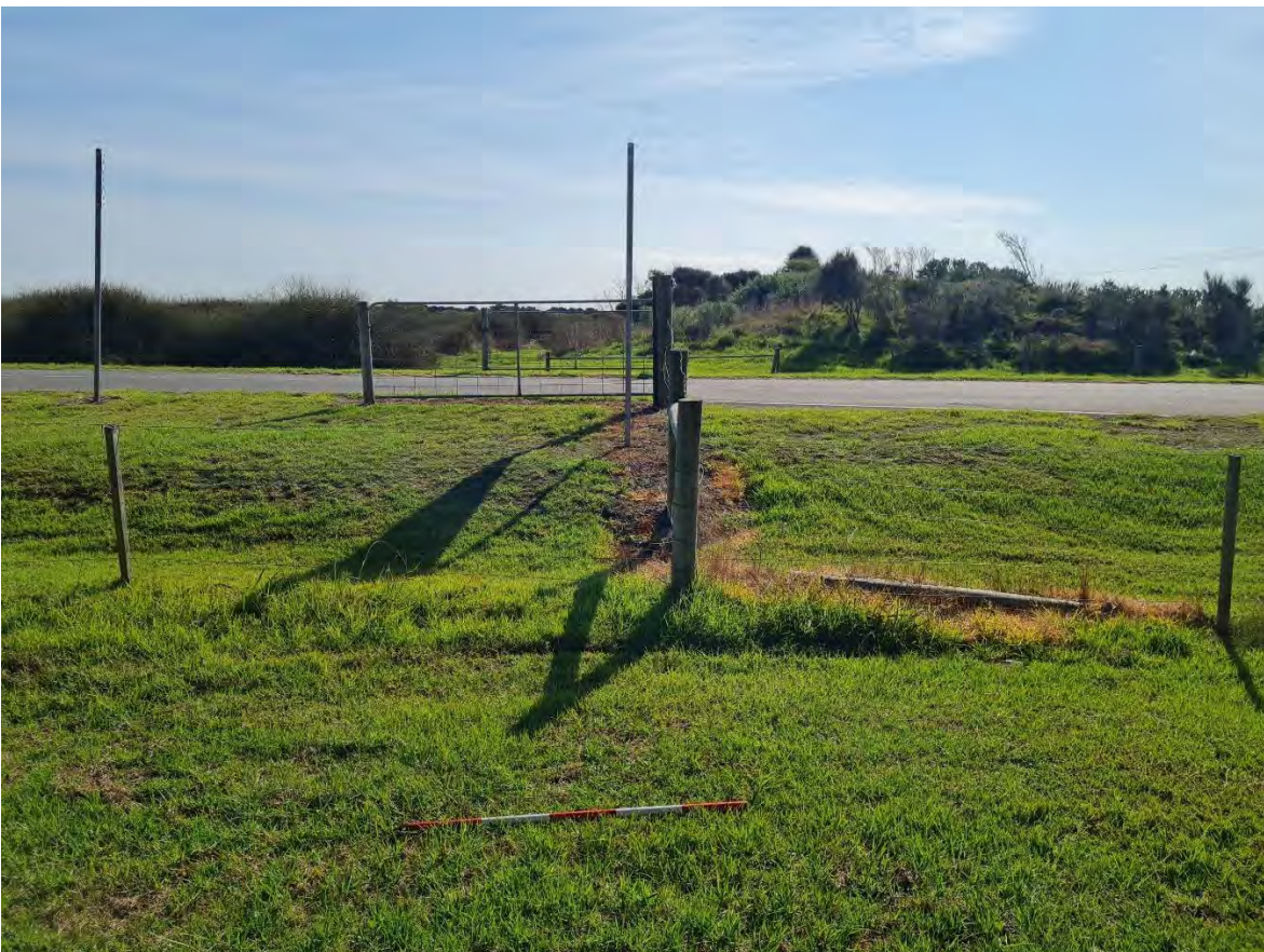
Plate 23 Southern access road, drainage and utilities, facing south (R. Stewart 26.04.2023)
