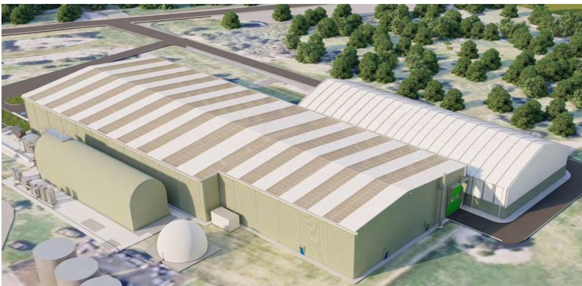
Figure 9 Warehouse building with nominated extent of skylight (3D render updated 23 rd of July 2024)
