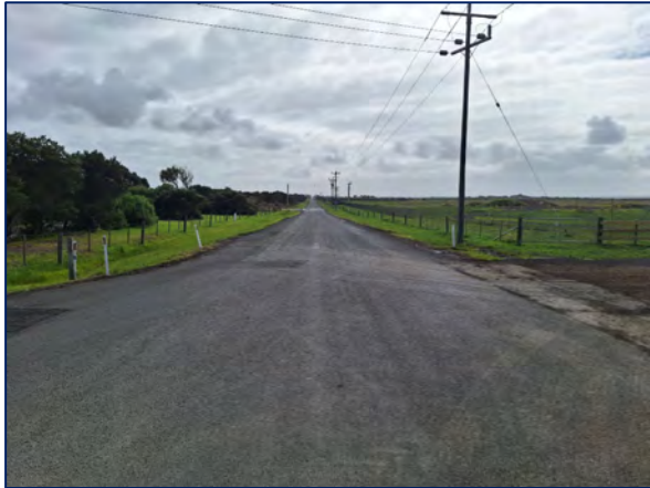
Figure 6: Blackrock Road - View North
