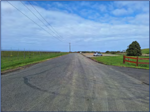
Figure 7: Blackrock Road - View South
