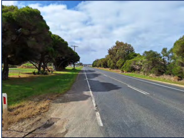
Figure 8: Barwon Heads Road - View East
