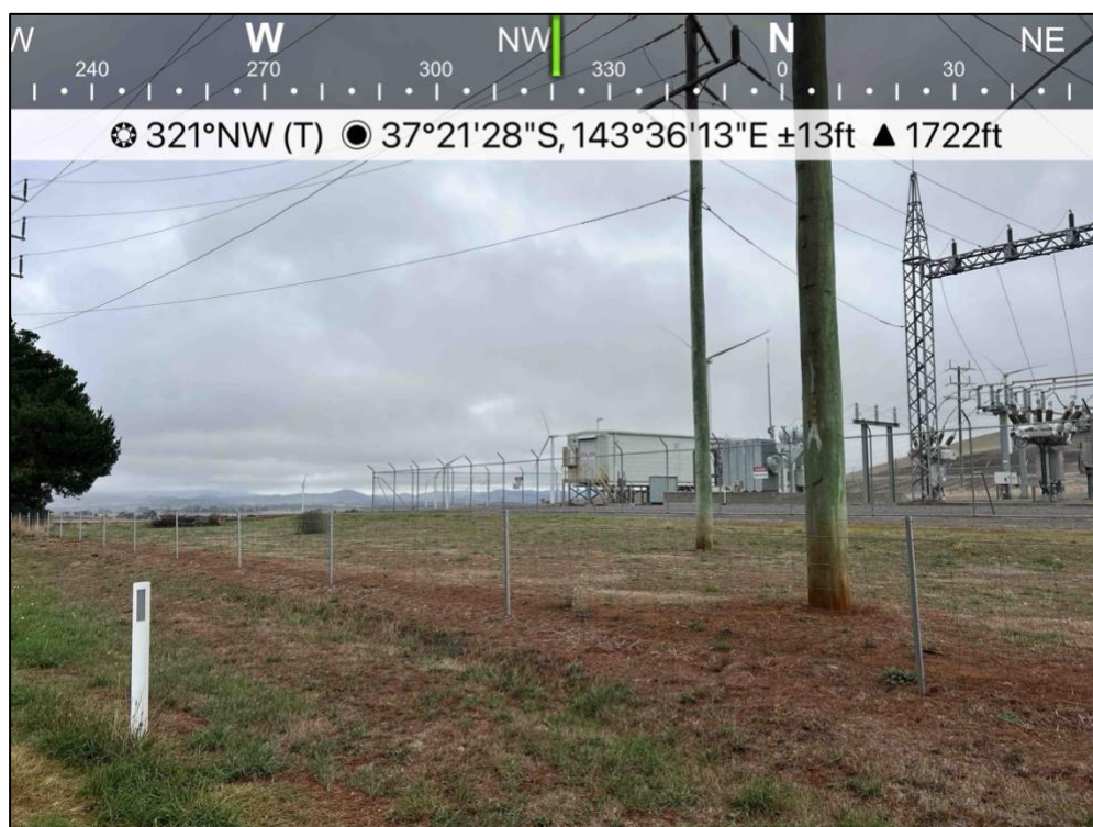
Figure 9 – Managed grass around and non-vegetated areas of the Waubra Wind Farm substation.
