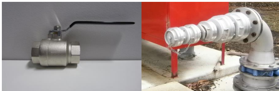
Image 1: 150 mm Full bore isolation valve (CFA, 2023).
