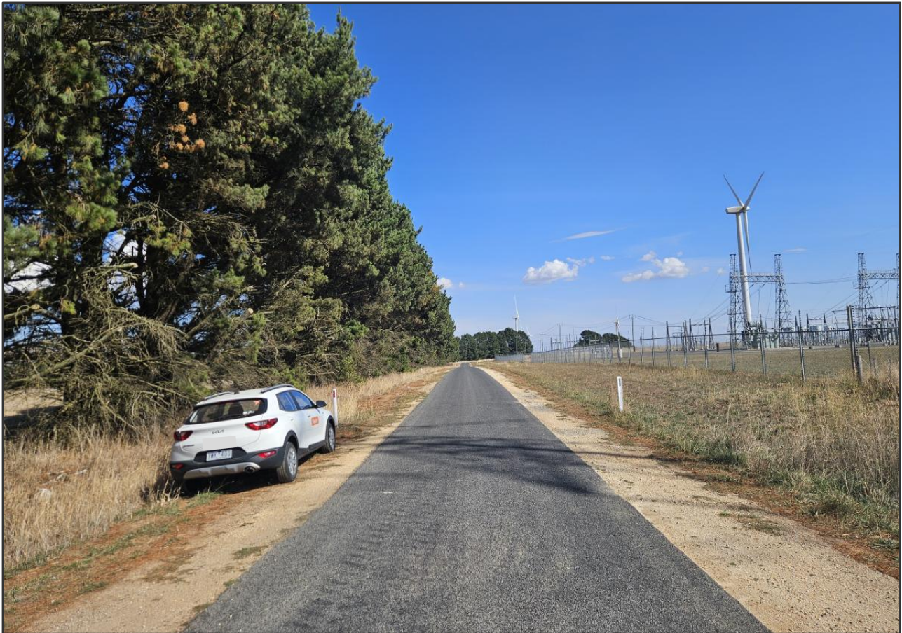
Figure 4 Troys Road, looking west adjacent to the subject site
