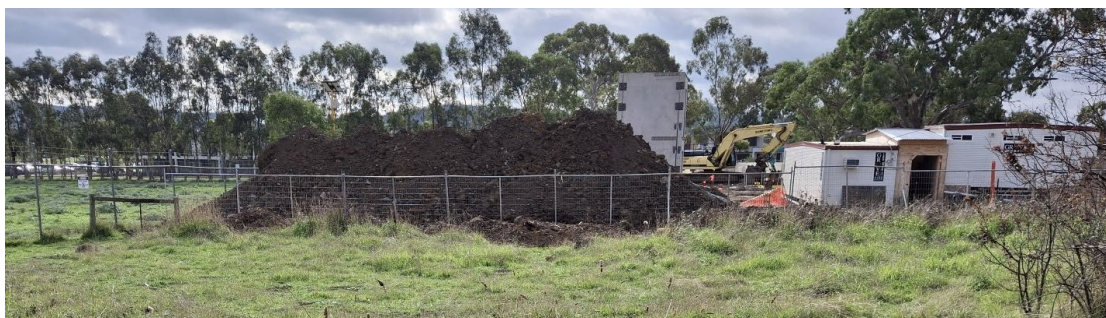
Image 35. Weedy north-west corner, showing proposed alignment for underground power and communications services in the adjoining land parcel currently used to stockpile soil (Abzeco 26/05/2026)
