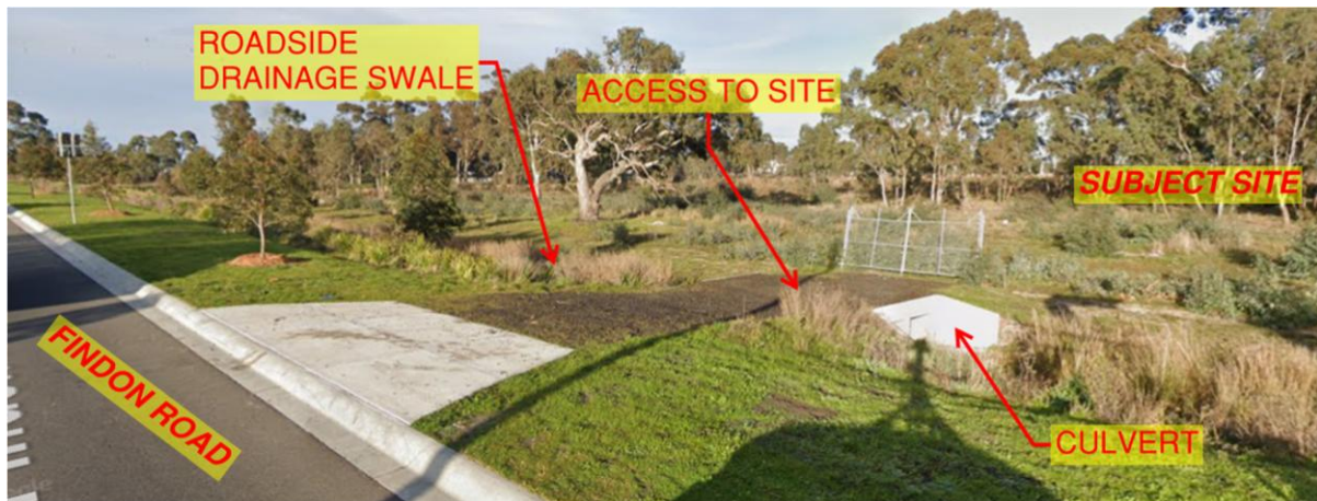
Fig.02: Adjacent Stormwater Infrastructure
