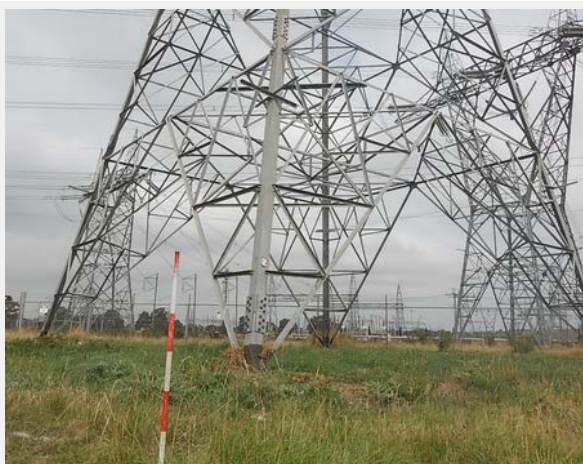
Photograph 9 Power tower in western extent of Activity Area indicating high disturbance, facing west (T. Fitzgerald 11/02/2020)
