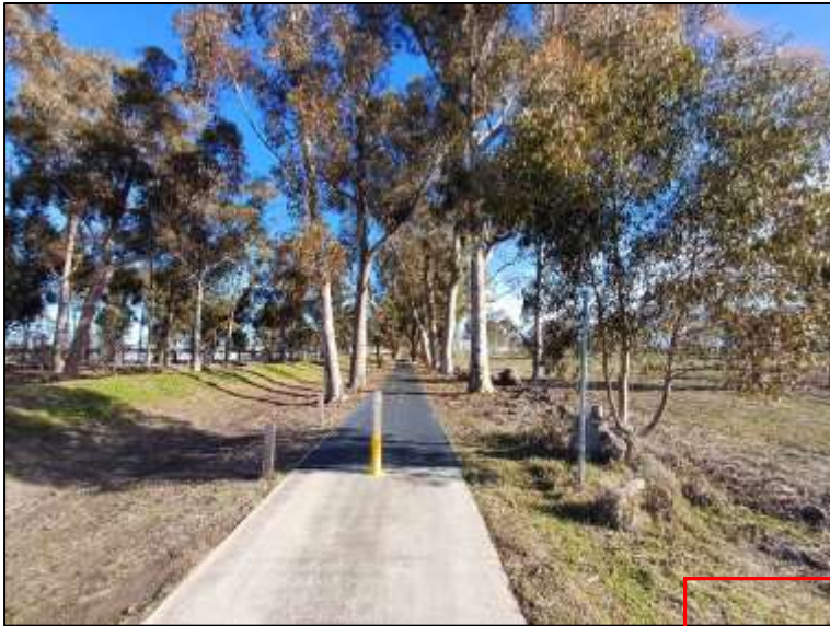
Pedestrian pathway as viewed from north east
