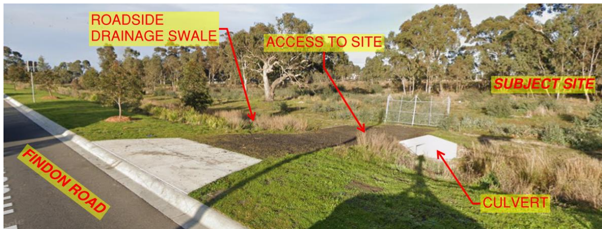
Fig.02: Adjacent Stormwater Infrastructure
