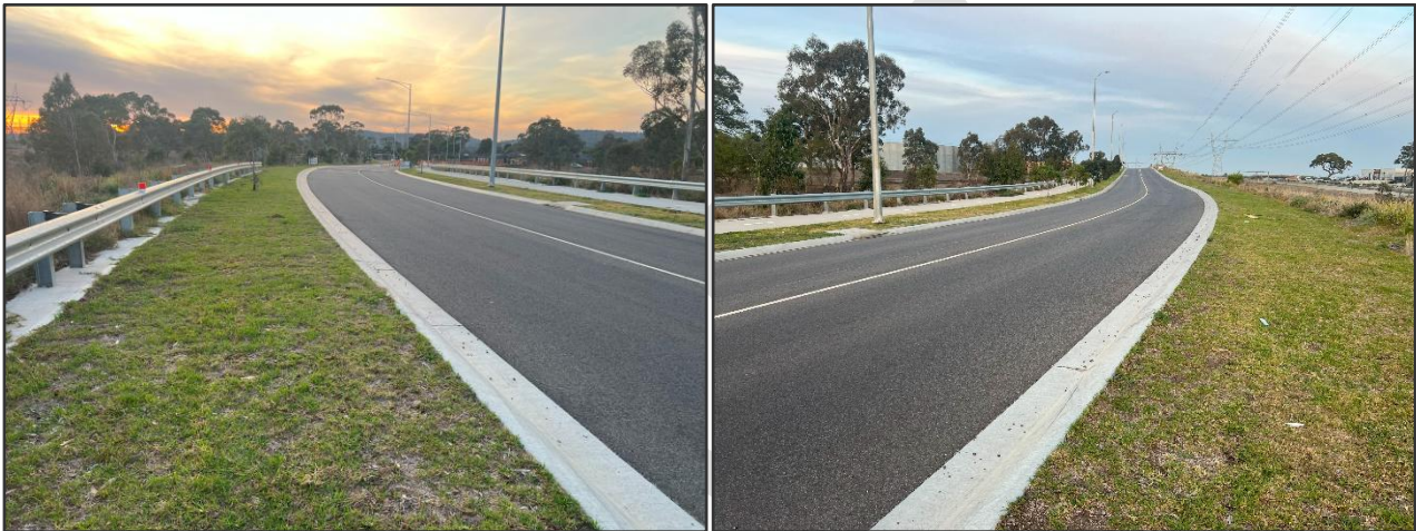
Figure 4 Findon Road looking Northwest (left) and Southeast (right) adjacent the Subject Site
