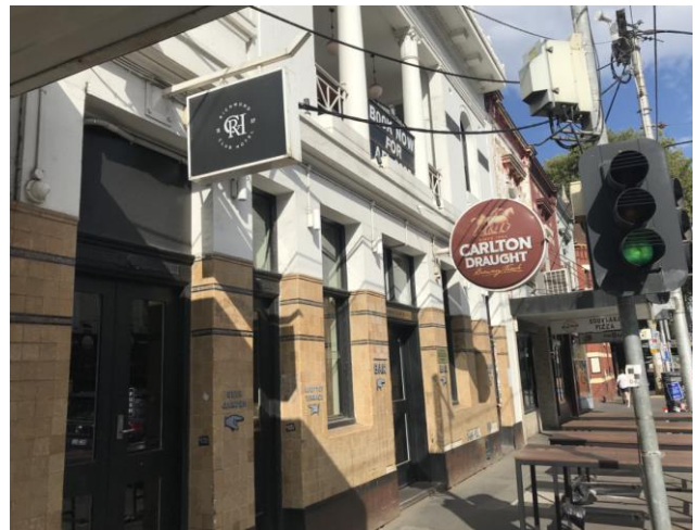
Figure 6 – The ground floor façade of the Richmond Club Hotel.
