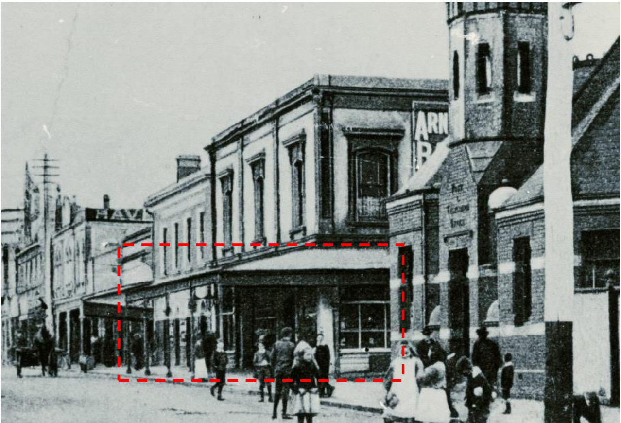
Figure 21 – Detail of Figure 20, showing the original return verandah to shopfronts at 94-98 Swan Street.
