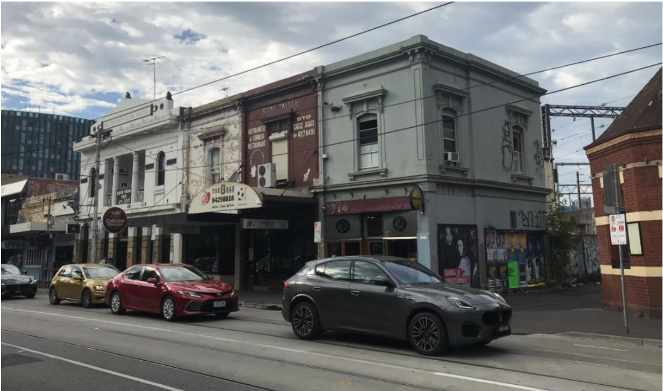
Figure 2 – The subject site viewed from the northwest across Swan Street.
