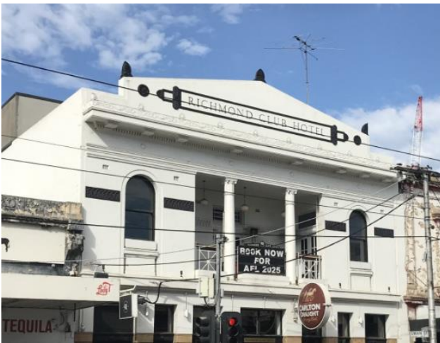
Figure 5 – The upper storey of the Richmond Club Hotel.
