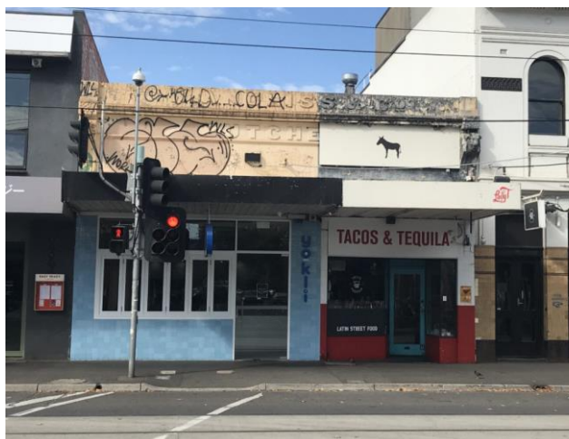
Figure 17 – The single storey shopfronts at 104-106 Swan Street, both graded contributory.
