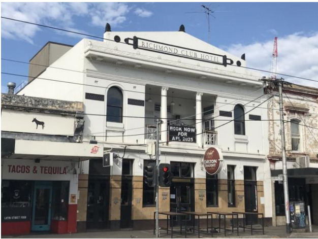
Figure 3 – The north Swan Street elevation of the Richmond Club Hotel.
