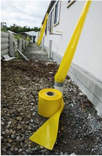
Figure A. Temporary downpipes (image credit: Northumberland Handyman Supplies Pty Ltd)
