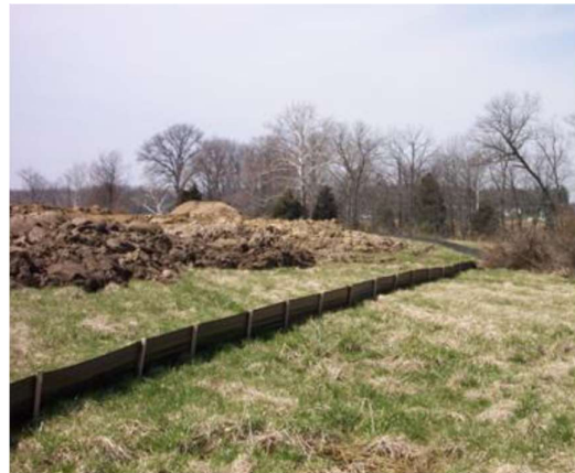
Figure D. Sediment trap (image credit: Delta T Solutions)
