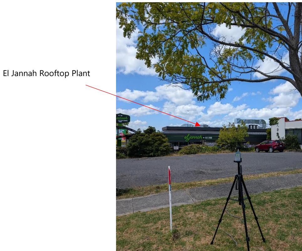
Image 2: View of El Jannah Rooftop plant to the northeast
