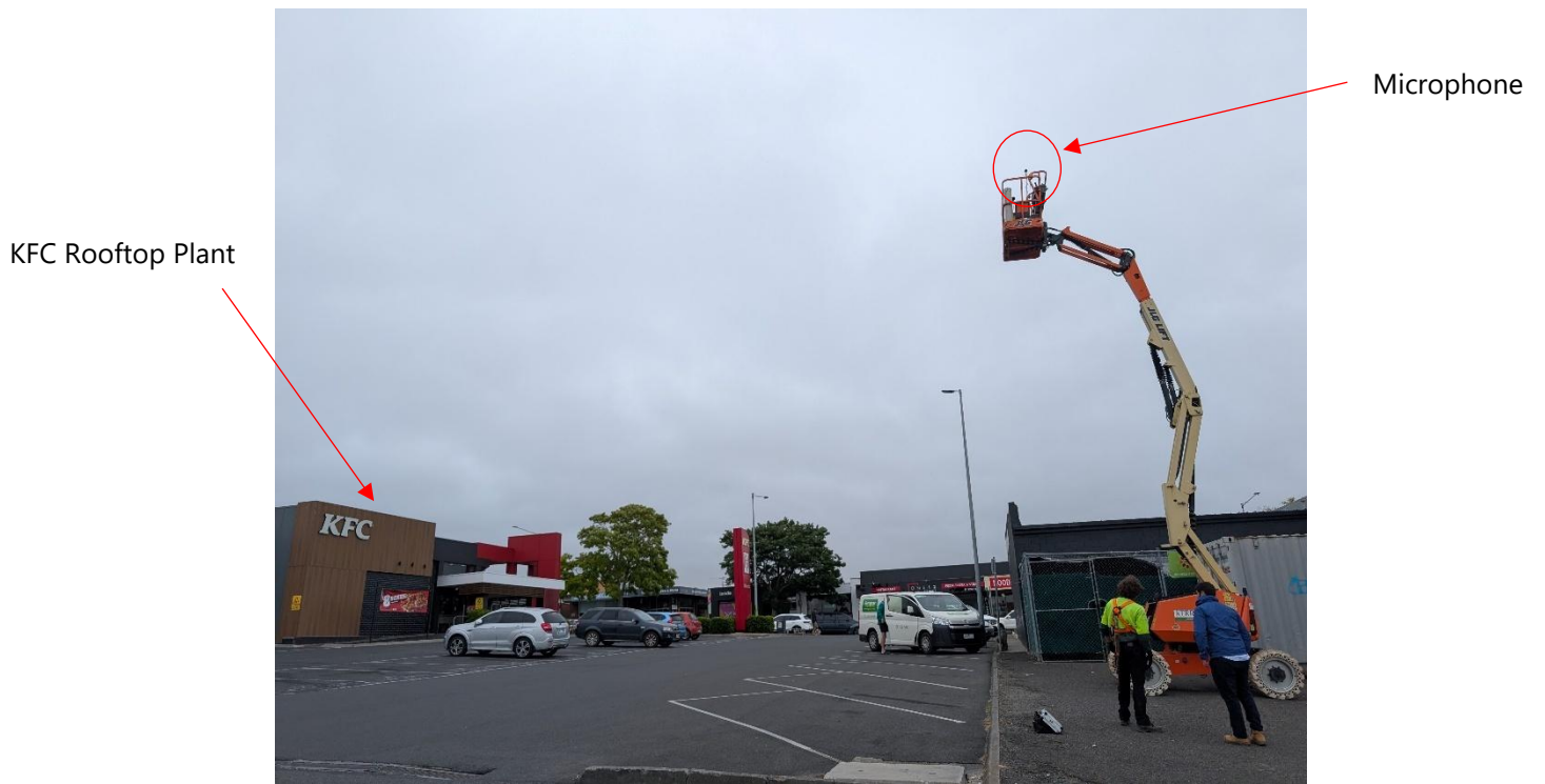
Image 1: Location B Unattended Monitor, Elevated on Boom Lift – View of KFC Rooftop plant
