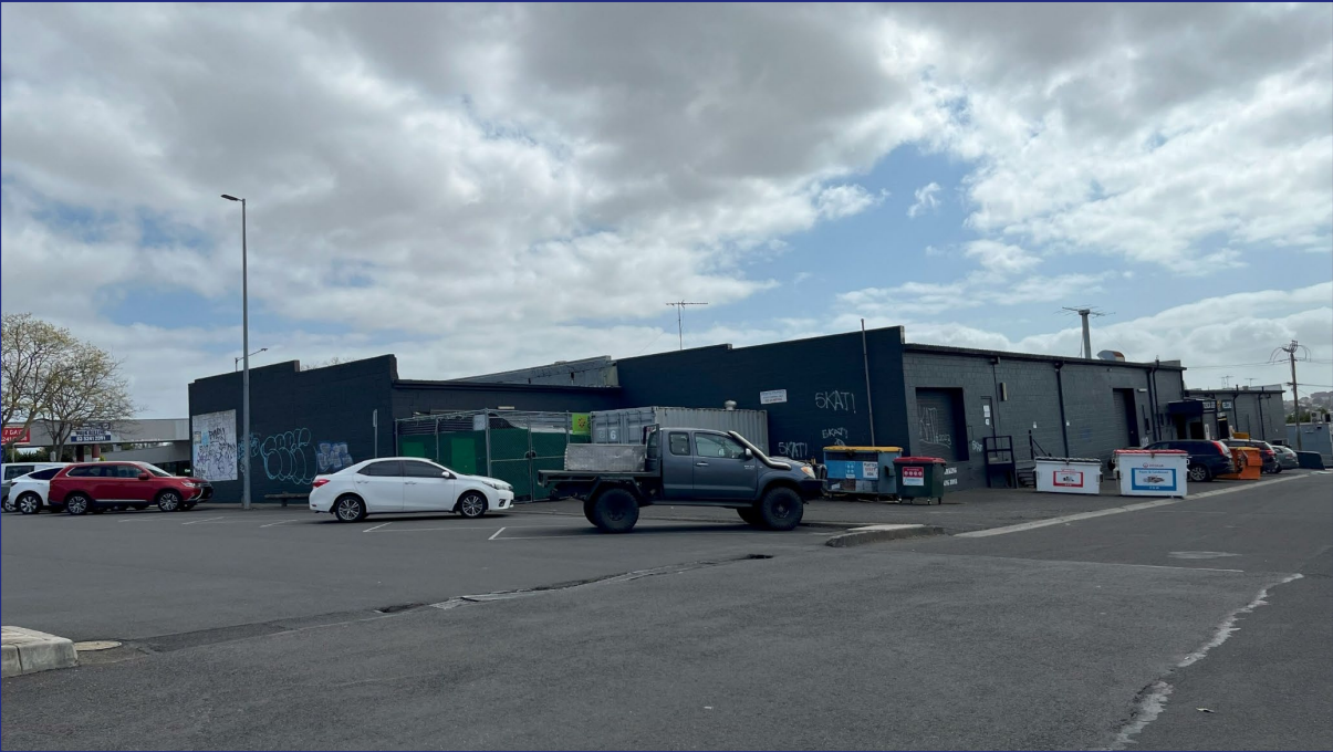
Figure 2: Subject Site – view north-west from Waterloo Street
