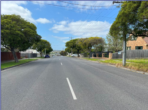
Figure 13: Regent Street – view south-east
