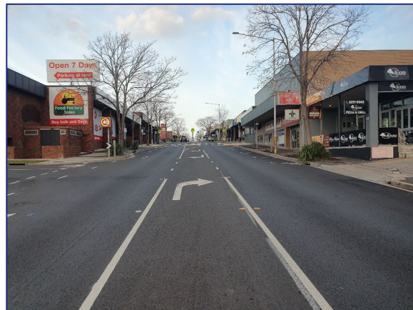
Figure 7: High Street – view south-west
