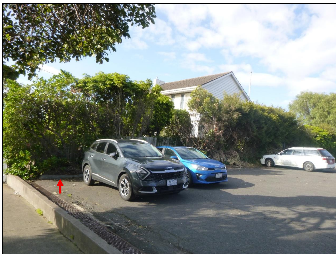
WYUNA PARADE. RAISED CARPARK AND DRAIN ADJACENT TO TREE 7. CONCRETE EDGING OF THE GARDEN ENCOMPASSES TREES 9, 10 AND 11.
