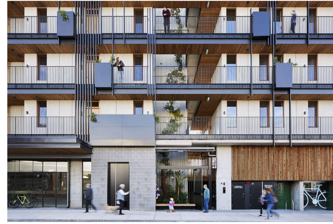
EXAMPLE PRECEDENT - OPEN AIR WALKWAY CORRIDOR PROJECT: NIGHTINGALE 2.0. ARCHITECT: SIX DEGREES ARCHITECTS. PHOTO: TESS KELLY.
