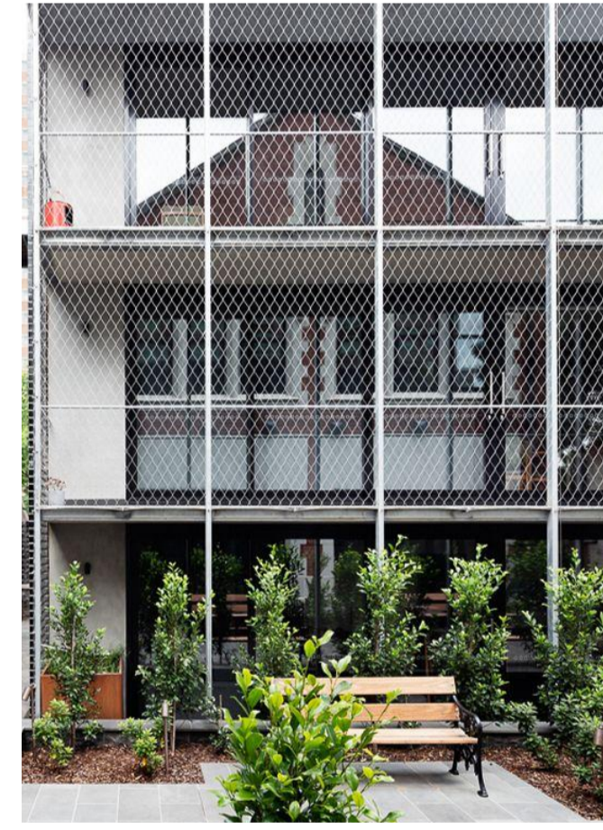
EXAMPLE PRECEDENT - OPEN AIR WALKWAY CORRIDOR MESH PROJECT: CHURCH ON NAPIER. ARCHITECT: KERSTIN THOMPSON. PHOTO: DYLAN JAMES.
