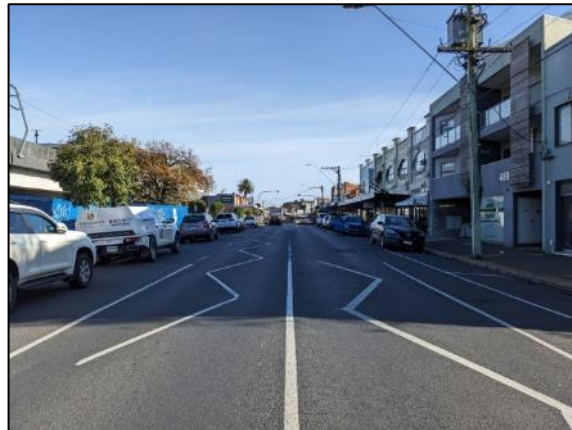
Figure 5: Neerim Road - View West
