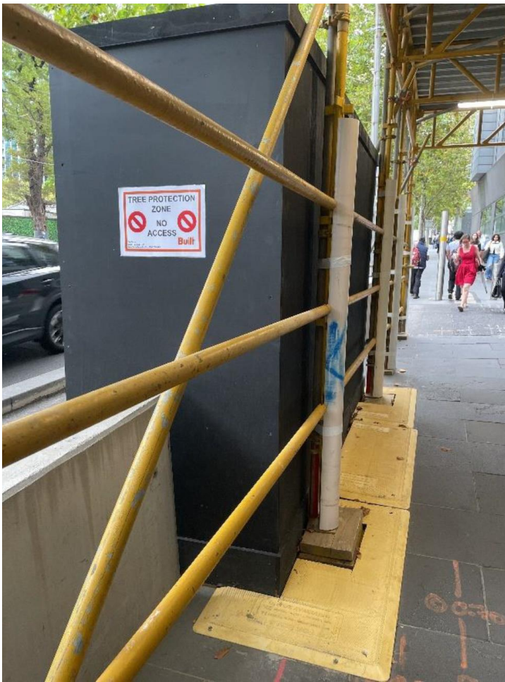
FIGURE 2 EXAMPLE TREE PROTECTION HOARDING
