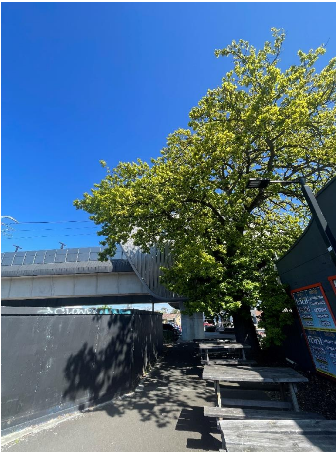
FIGURE 1 EXISTING HOARDING TO BE MAINTAINED FOR THE DURATION OF WORKS ADJACENT TO TREE 1
