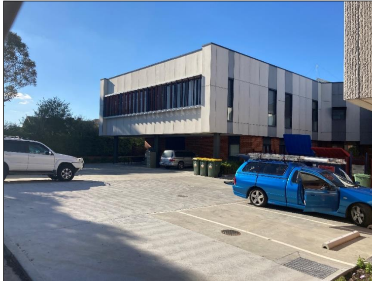
Figure 4: Secondary On-site Staff Car Parking Area, accessed from Graham Place (14 spaces)
