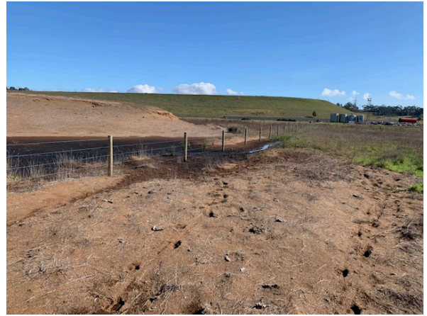
Figure 2-8: Stockpiling southwest extent of Project area – view west
