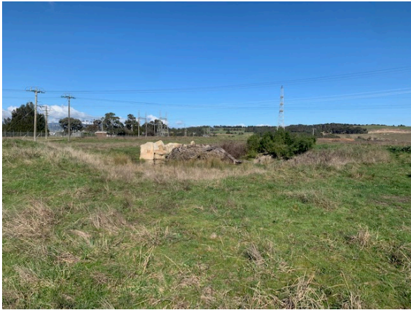
Figure 2-7: Dam in middle of Project area – view south
