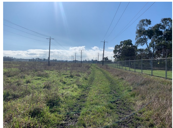
Figure 2-4: Access track along fence line of MWTS - view north
