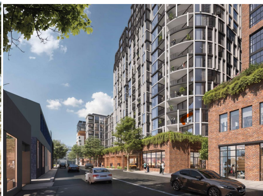
Figure 7 -Tower B (and C) Doonside Street
