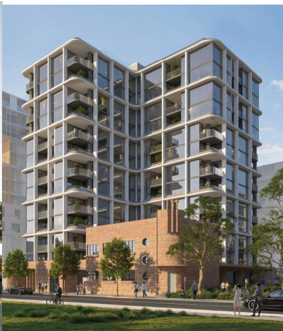
Figure 9 - Tower C – Doonside Street
