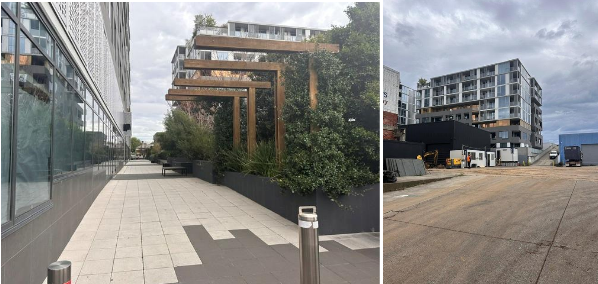
Figure 12 and 13 - Walkway through the Embassy Apartments, view of the Embassy apartments to the rear of future Building C.
