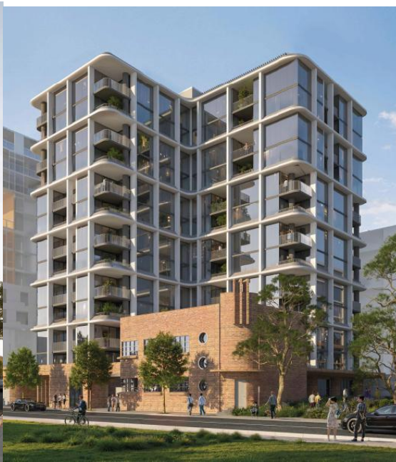
Figure 9 - Tower C – Doonside Street
