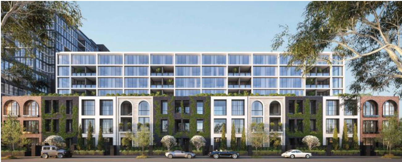
Figure 10 - Building D – Appleton Street.
