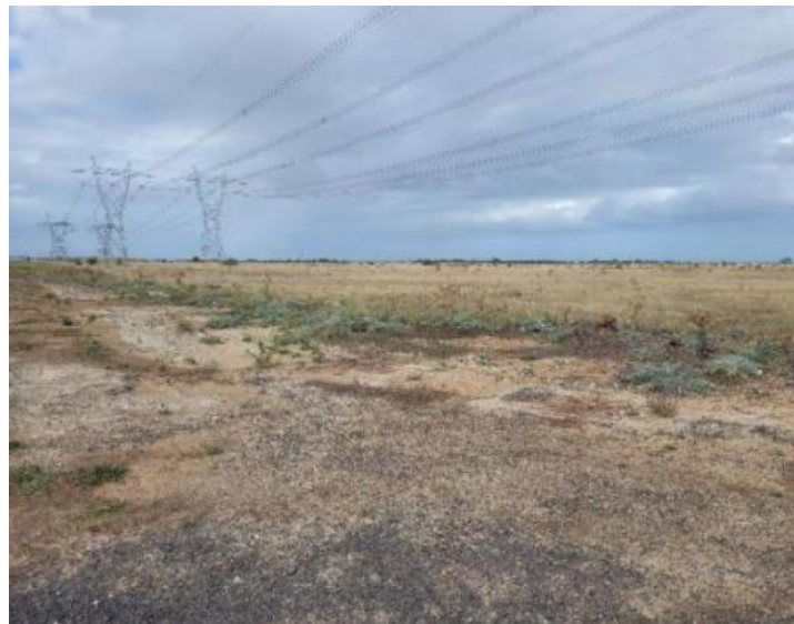
Figure 16 – Transmission lines south of the site within easement (Source: Application)
