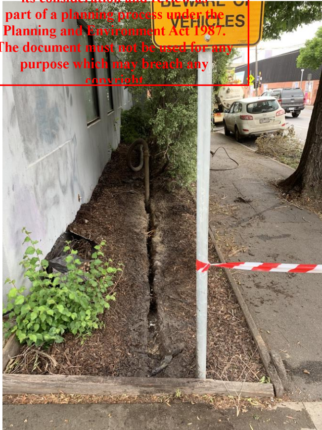
Contextual view of the trench and elm trunk.
