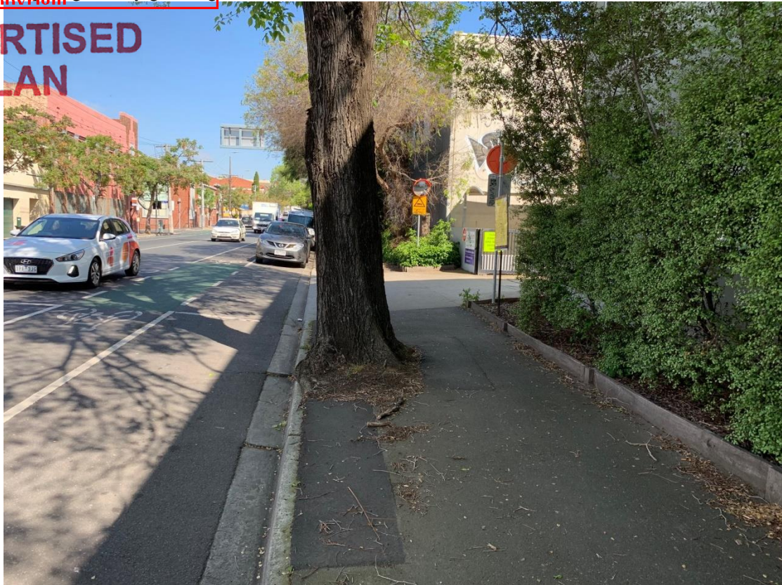
Tree 1, looking west – lean over the road is obvious.
