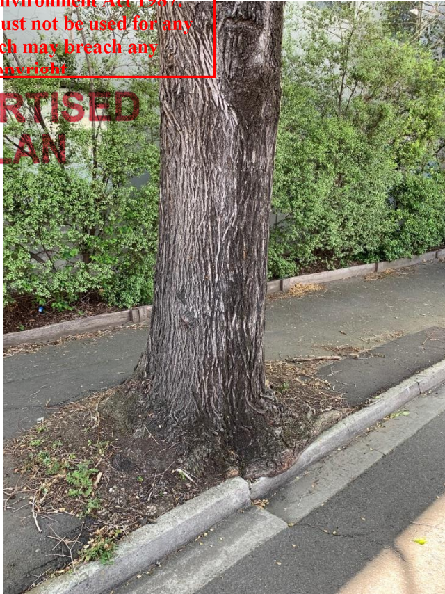
View of structural damage and encroachment of the trunk over the kerb.
