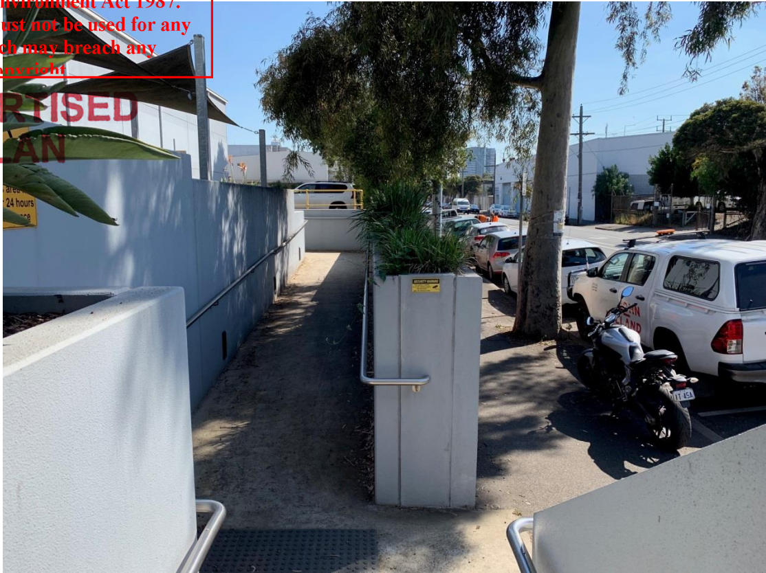
Significant root development is highly unlikely beneath the pedestrian concrete ramp opposite tree 5. Excavation to the left of the planter can take place without harming the tree.
