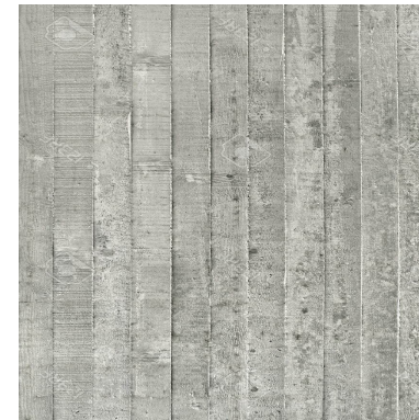
CN05 - BOARD FORMED PRECAST CONCRETE
