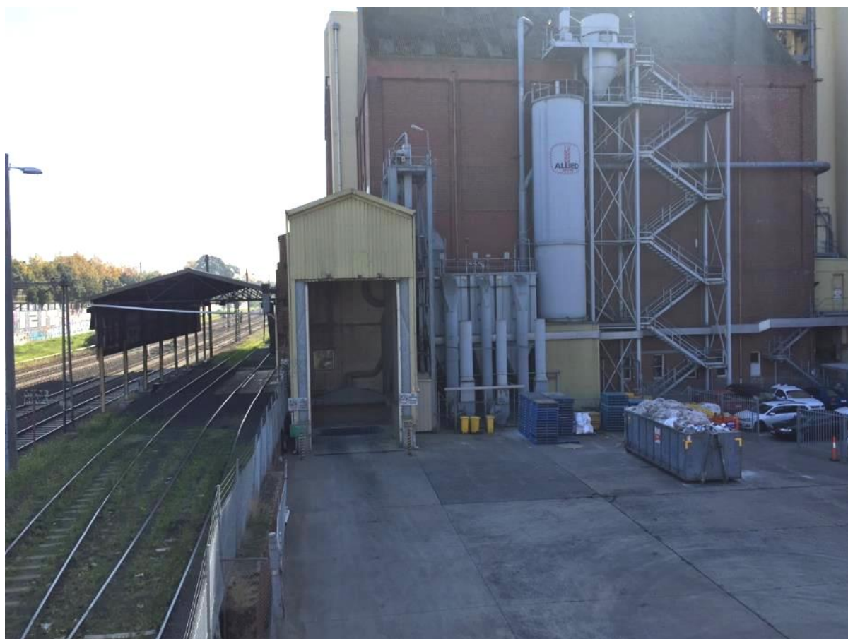
Figure 4: Truck and rail unloading facilities. Photographed 16/5/17.
