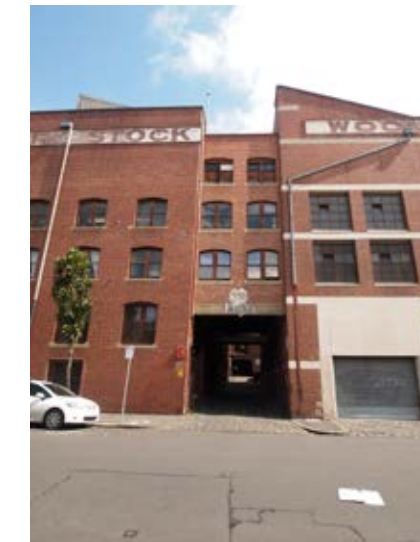
04 View of existing Building 'S3' undercroft entry
