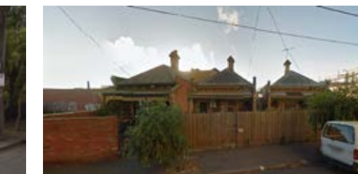
03 RESIDENTIAL 31-35 ELIZABETH ST- ONE STOREY
