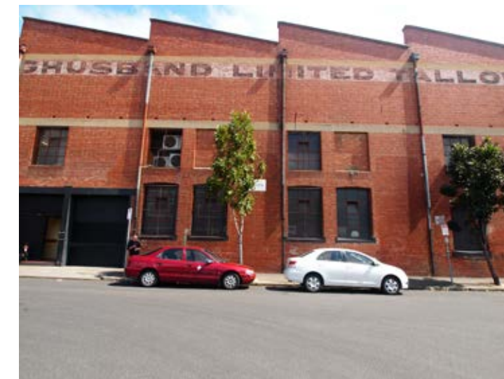
03 Partial view of existing Building 'S3' Elizabeth Street facade All historical signage to remain
