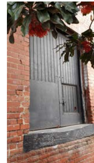
05 View of existing Building 'S3' 'S3' loading door to remain
