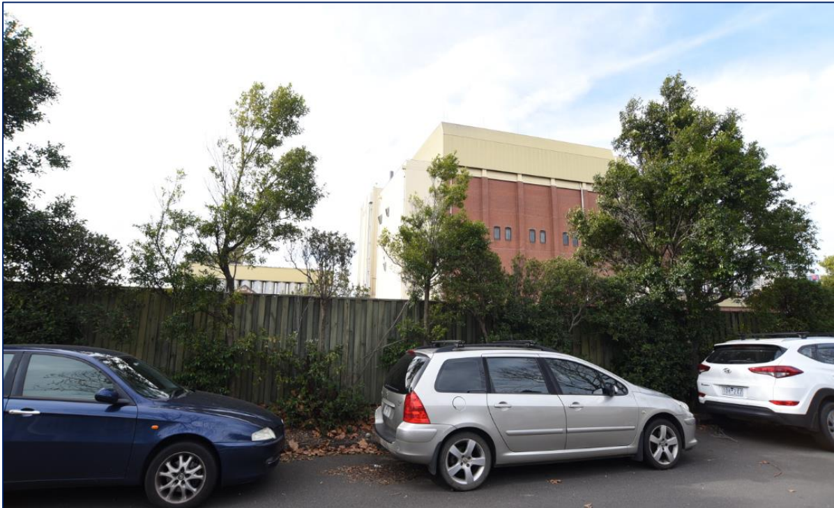
Photo 10: Looking east from Bellair Street across the railway reserve with the Allied Pinnacle buildings in the background.
