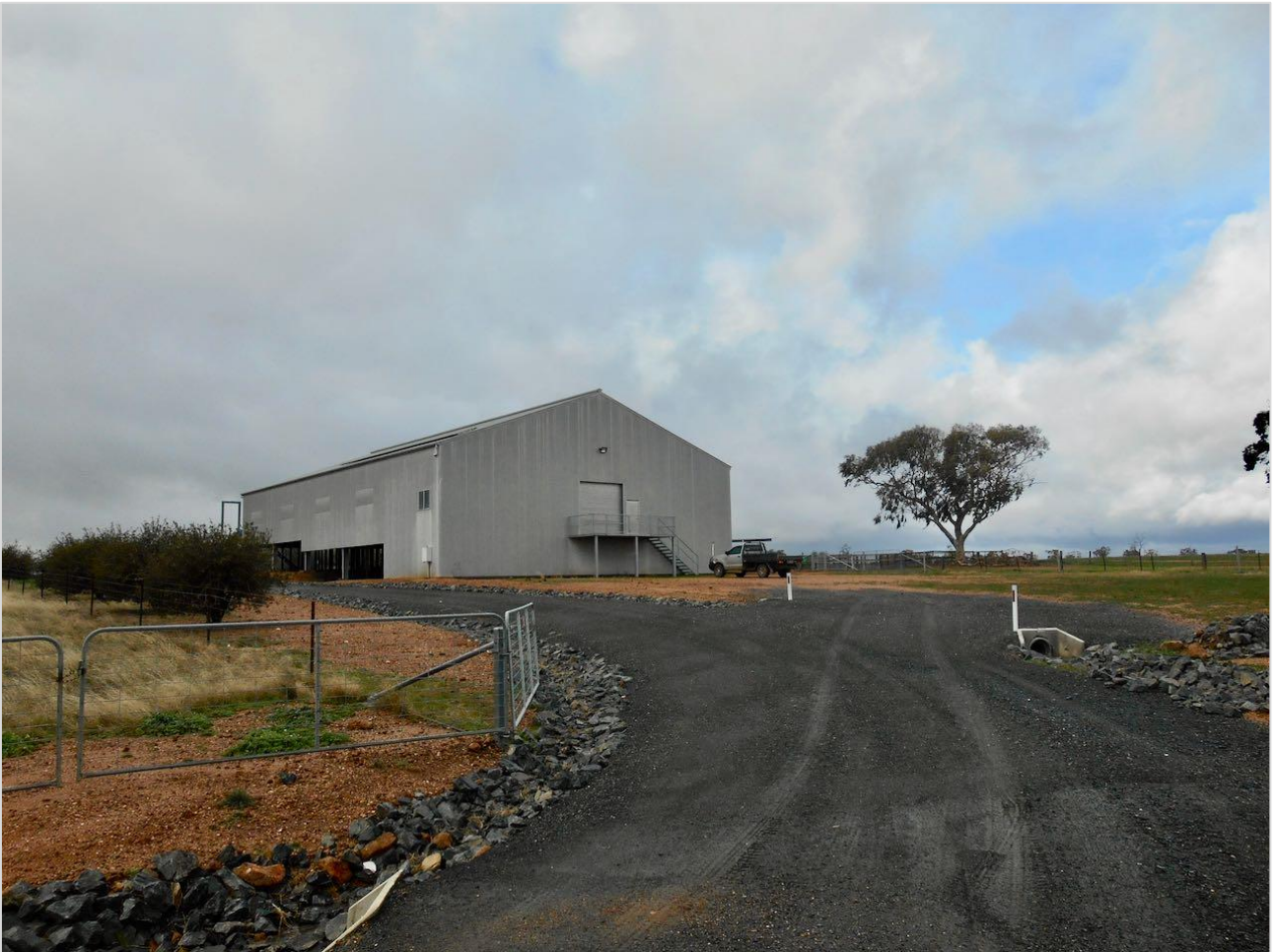
Figure 3-2: Shearing shed located near the BESS site
